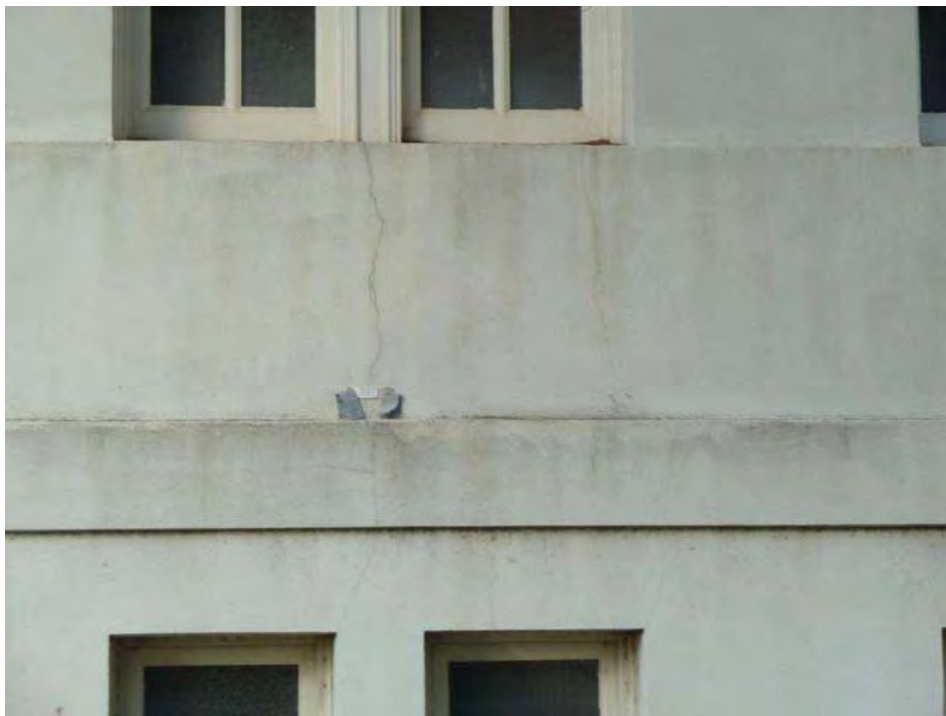
13th Street and Lakeside (close up of above): cracked wall, peeling paint.
