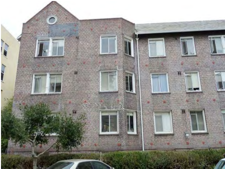
Bay Place and Access Road: partially reinforced masonry building vulnerable to serious damage from seismic events, cracked masonry wall potentially hazardous in event of earthquake.
