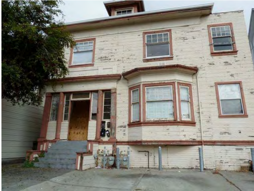
26th Street and Telegraph: serious deterioration apparently due to long-term neglect, boarded door, peeling paint, dry rot.
