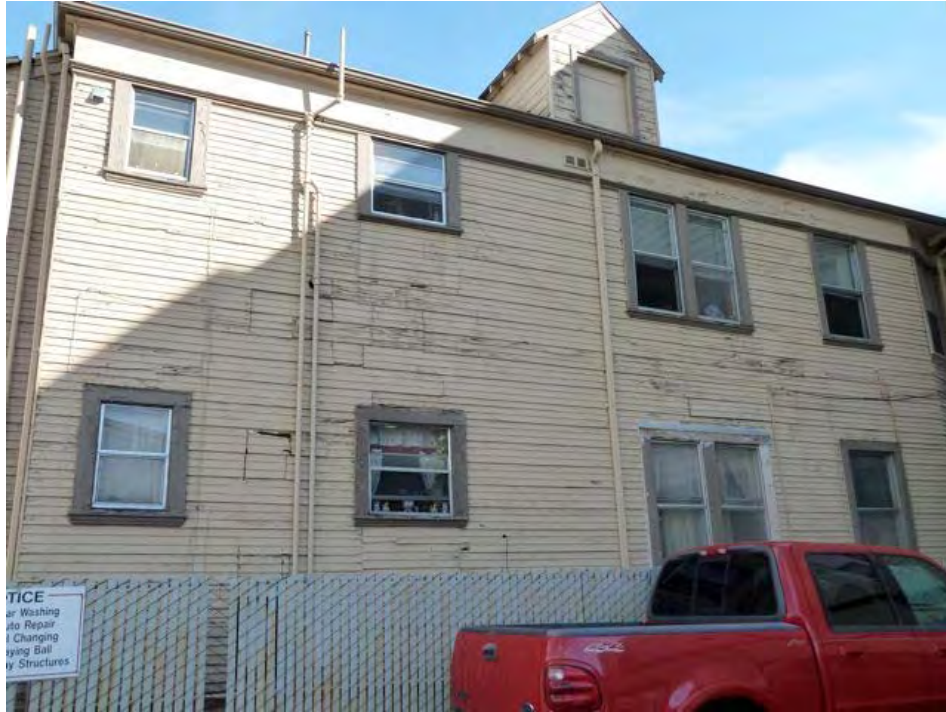
14th Street and Castro: serious deterioration apparently due to long-term neglect, missing siding, peeling paint, dry rot.
