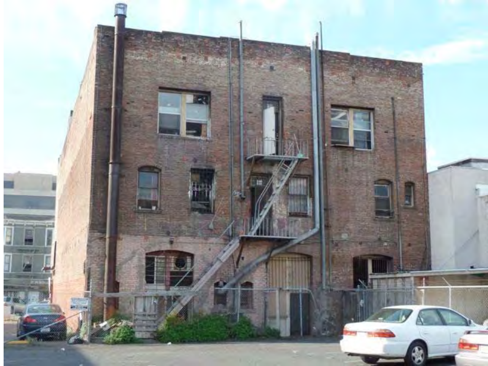
8th Street and Clay: partially reinforced masonry building vulnerable to serious damage from seismic events, cracked wall potentially hazardous in event of earthquake, serious deterioration and dilapidation due to apparent long-term neglect.
