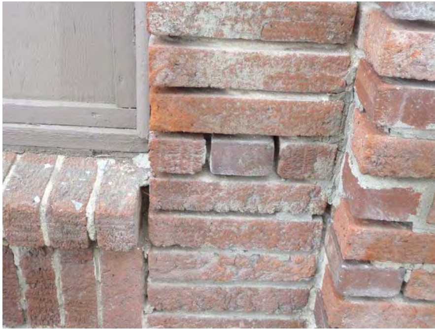
23rd Street and Valley: deteriorated masonry wall potentially hazardous in event of earthquake, building vulnerable to serious damage from seismic events.
