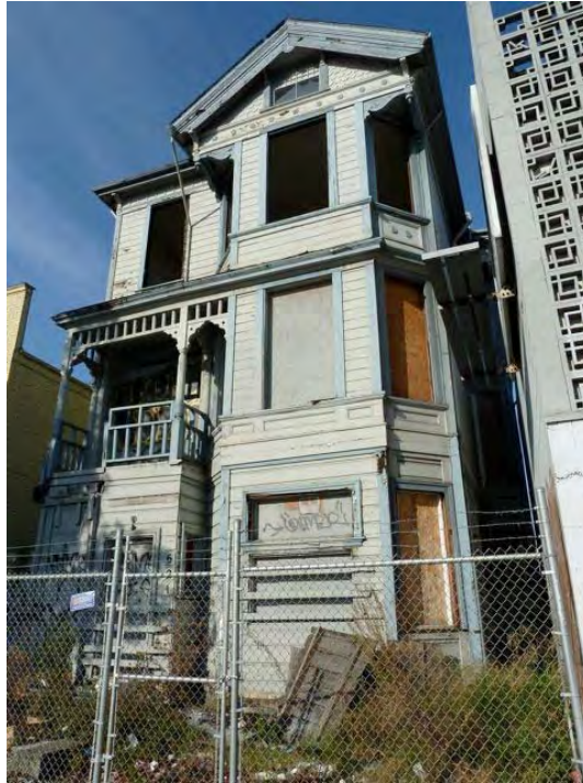
7th Street and Harrison: serious deterioration apparently due to long-term neglect, peeling paint, missing and boarded windows, dry rot.
