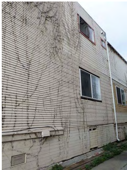
26th Street and Telegraph: deteriorated siding, cracked foundation and peeling paint apparently due to long-term neglect.
