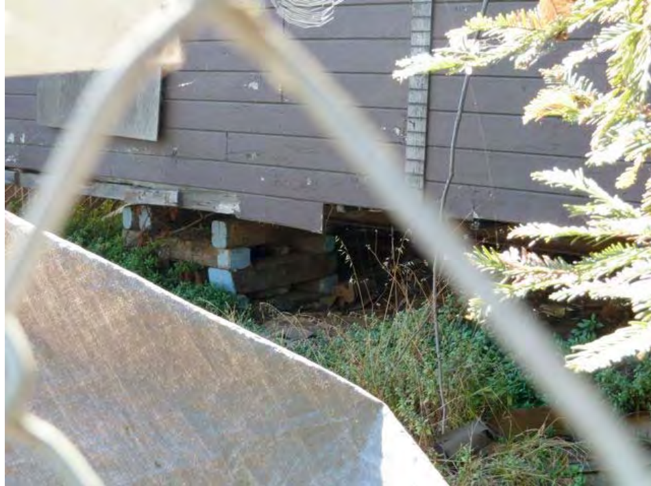
5th Street and Brush: vulnerable to serious damage from seismic hazards due to lack of foundation.
