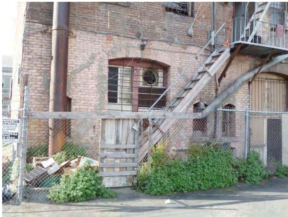
8th Street and Clay (close up of above): extensive cracked masonry wall potentially hazardous in event of earthquake, building vulnerable to serious damage from seismic events.
