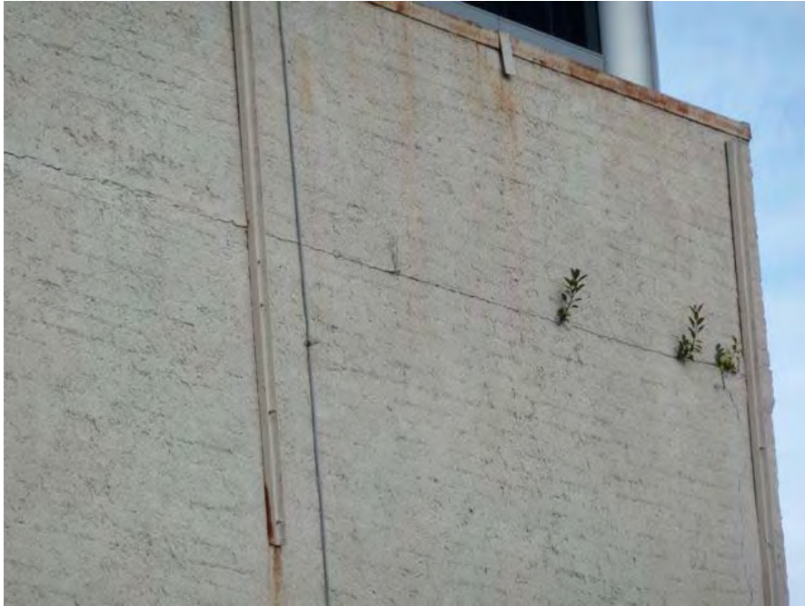
Grand and Valdez: unreinforced masonry building vulnerable to serious damage from seismic events, cracked masonry wall potentially hazardous in event of earthquake.
