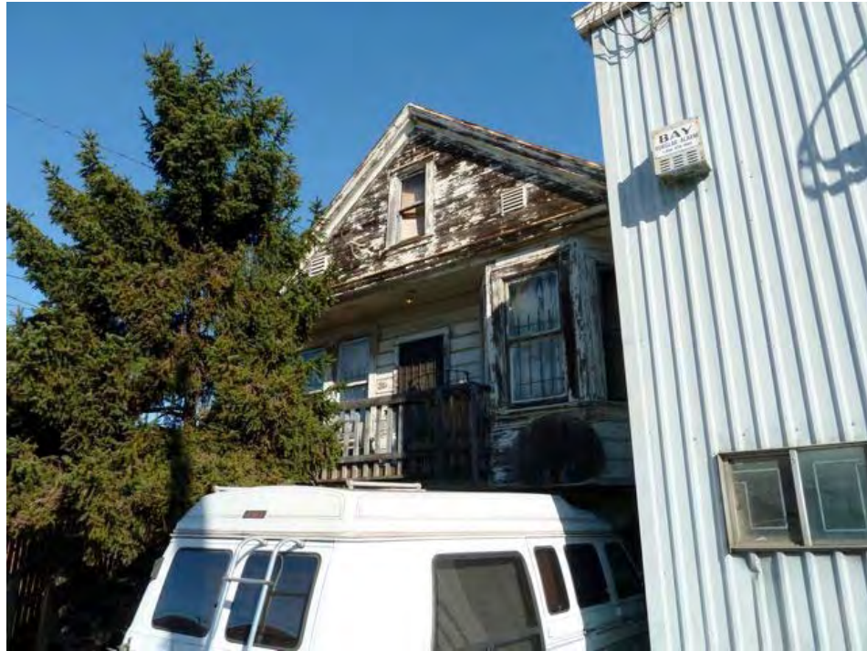
4th Street and Brush: serious deterioration and dilapidation apparently due to long-term neglect, deteriorated siding and eaves, peeling paint, dry rot.
