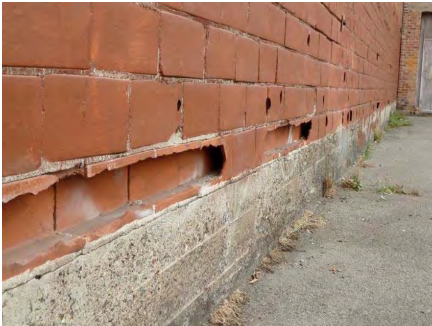
24th Street and Valley (same building as previous photo): deteriorated and missing masonry potentially hazardous in event of earthquake, building vulnerable to serious damage from seismic events.
