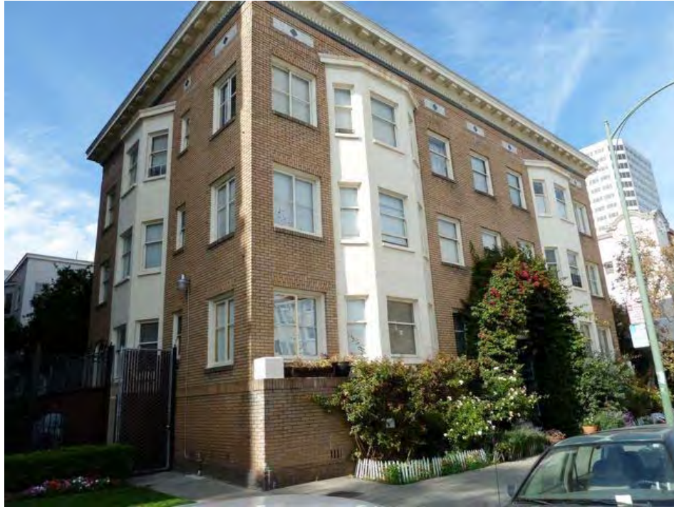
17th Street and Alice: masonry building vulnerable to serious damage from seismic events, building potentially hazardous in event of earthquake.
