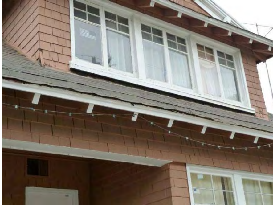
24th Street and Waverly: deteriorated roof apparently due to long-term neglect.
