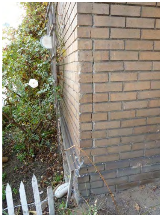
17th Street and Alice (close up of above): cracked masonry at building corner potentially hazardous in event of earthquake, building vulnerable to serious damage in event of earthquake.
