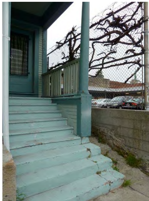
24th Street and Valdez (close up of above): cracked stairs, peeling paint, dry rot.
