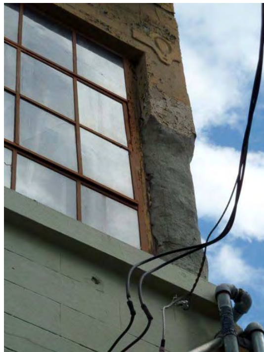
3rd Street and Broadway: dry rot, peeling paint, deteriorated wall.
