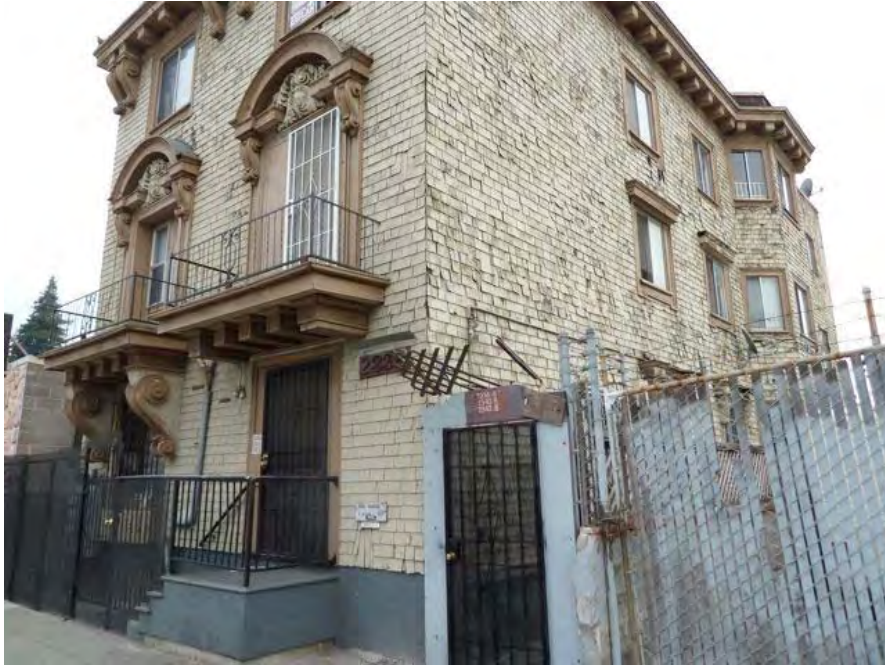
24th Street and Telegraph: serious deterioration and dilapidation apparently due to long-term neglect, deteriorated siding, dry rot, peeling paint.
