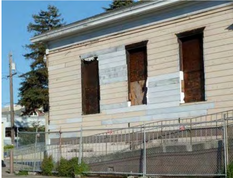
7th Street and Martin Luther King: serious deterioration apparently due to long-term neglect, missing and boarded windows, peeling paint, deteriorated siding.
