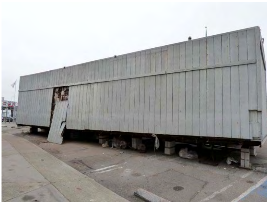
27th Street and Broadway (same building as previous photo): severely deteriorated walls likely allowing moisture intrusion, mold contamination and structural wood rot. Potentially unsafe pier foundation.
