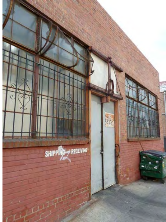
9th Street and Clay: unreinforced masonry building vulnerable to serious damage from seismic events, potentially hazardous in event of earthquake, deteriorated facade, graffiti.
