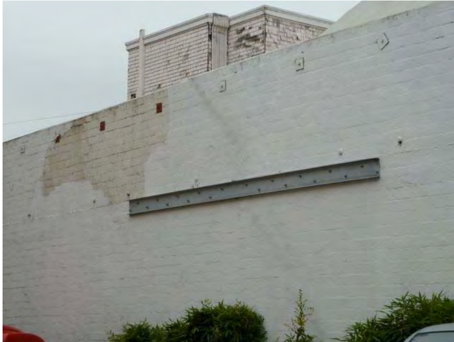
24th Street and Harrison: partially reinforced building vulnerable to serious damage from seismic events, cracked masonry wall potentially hazardous in event of earthquake.
