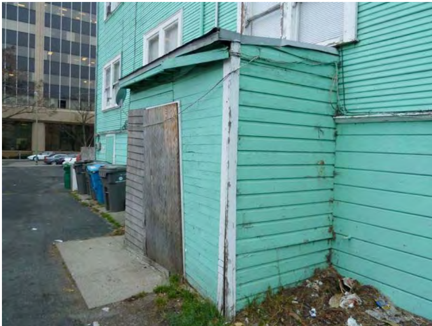
23rd Street and Waverly: deteriorated siding, peeling paint, dry rot, and boarded doors apparently due to long-term neglect.
