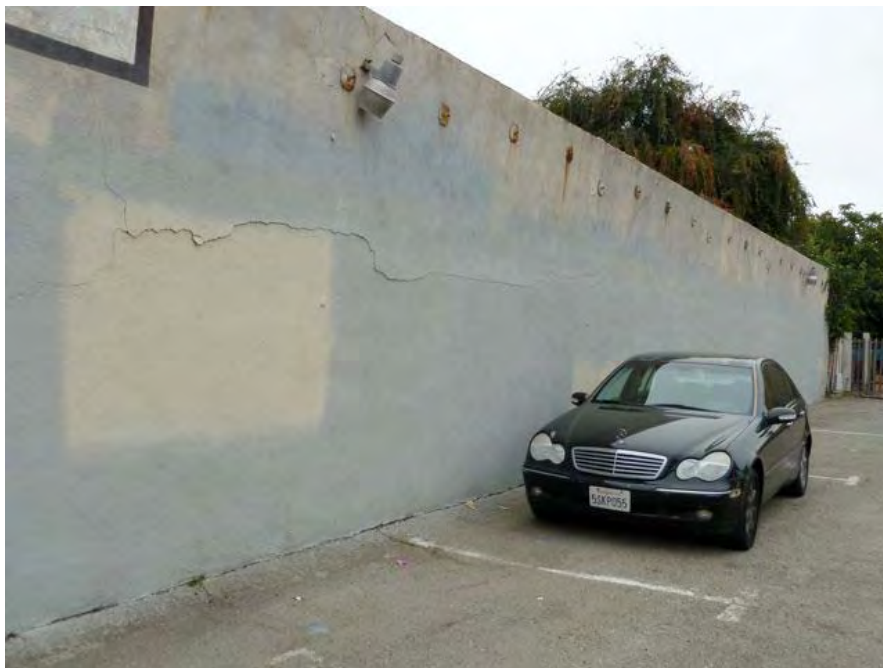
24th Street and Valdez: partially reinforced masonry building vulnerable to serious damage from seismic events, cracked wall potentially hazardous in event of earthquake.
