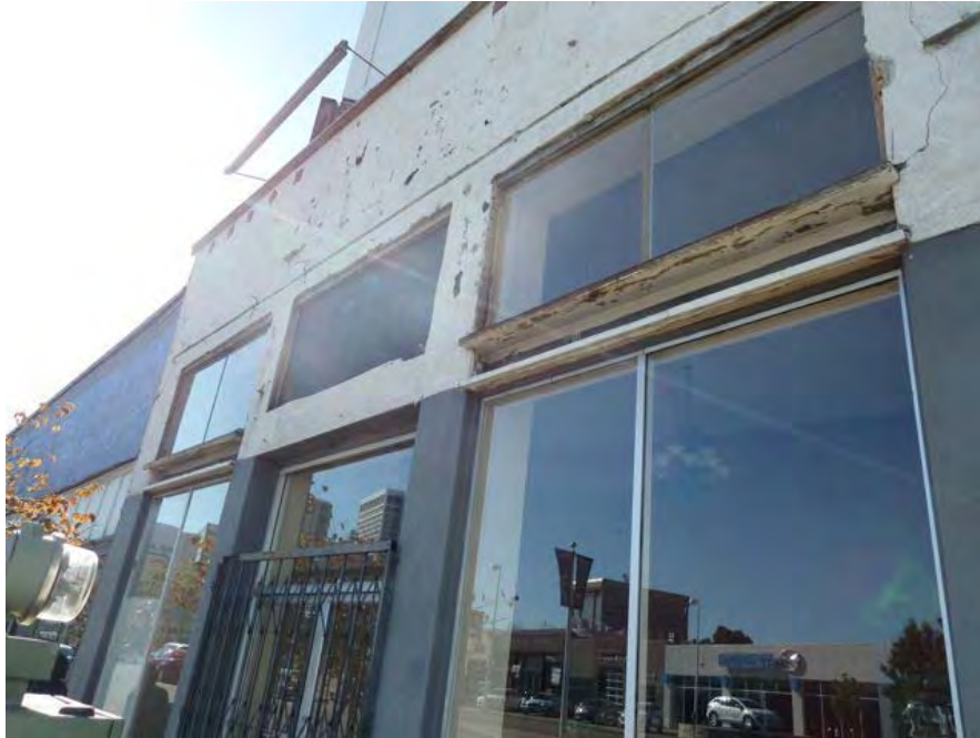
26th and Broadway: peeling paint, dry rot and cracked wall on commercial building apparently due to long-term neglect.
