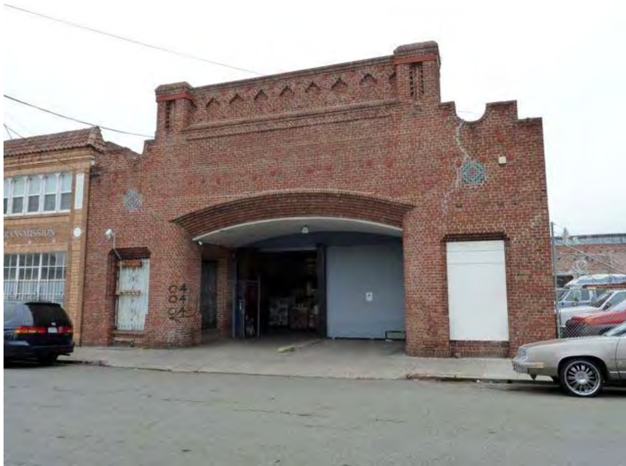
24th Street and Valley: partially reinforced masonry building vulnerable to serious damage from seismic events, cracked wall potentially hazardous in event of earthquake, boarded windows.
