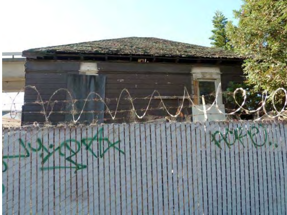
5th Street and Brush: serious dilapidation apparently caused by long-term neglect, missing and boarded windows, deteriorated siding, severe roofing dilapidation likely allowing moisture intrusion, mold contamination and structural wood rot.
