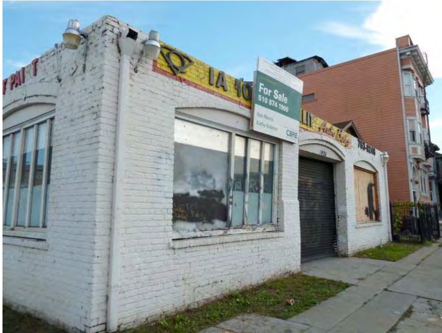
20th Street and Castro: partially reinforced masonry building vulnerable to serious damage from seismic events, potentially hazardous in event of earthquake, vacant and boarded commercial building, graffiti.
