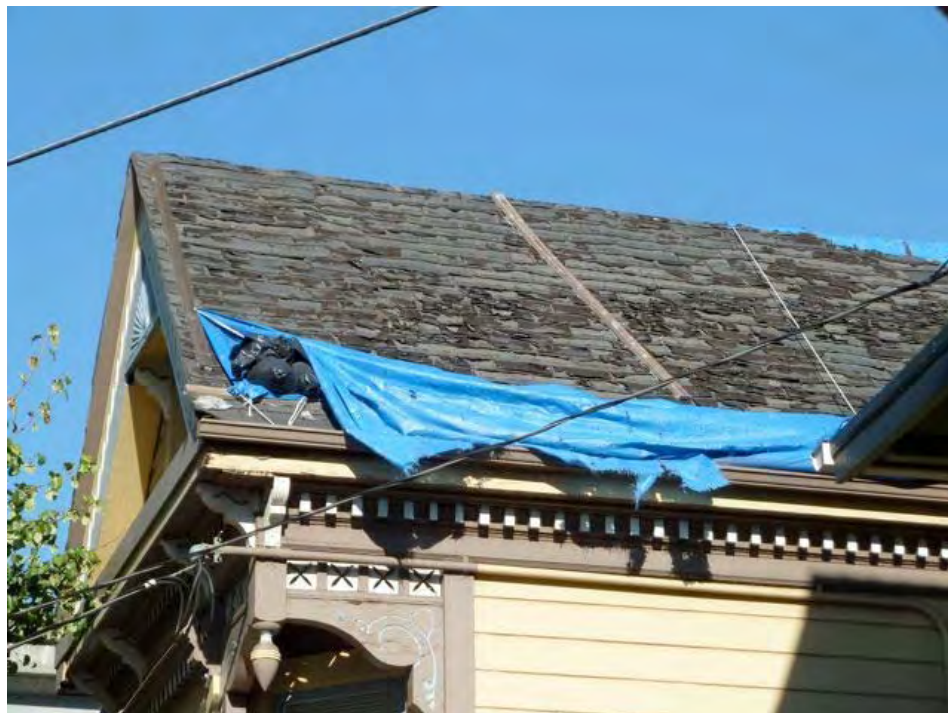
4th Street and Jefferson: severe roof dilapidation likely allowing moisture intrusion, mold contamination and structural wood rot.
