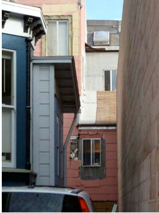
9th Street and Jefferson: deteriorated siding and roof likely allowing moisture intrusion, mold contamination and structural wood rot.
