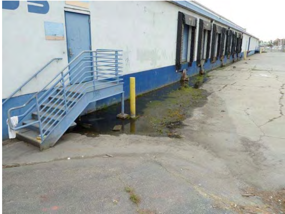
1st Street near Estuary Park (same building as previous photo): standing water caused by poorly constructed paved lot, cracked pavement.
