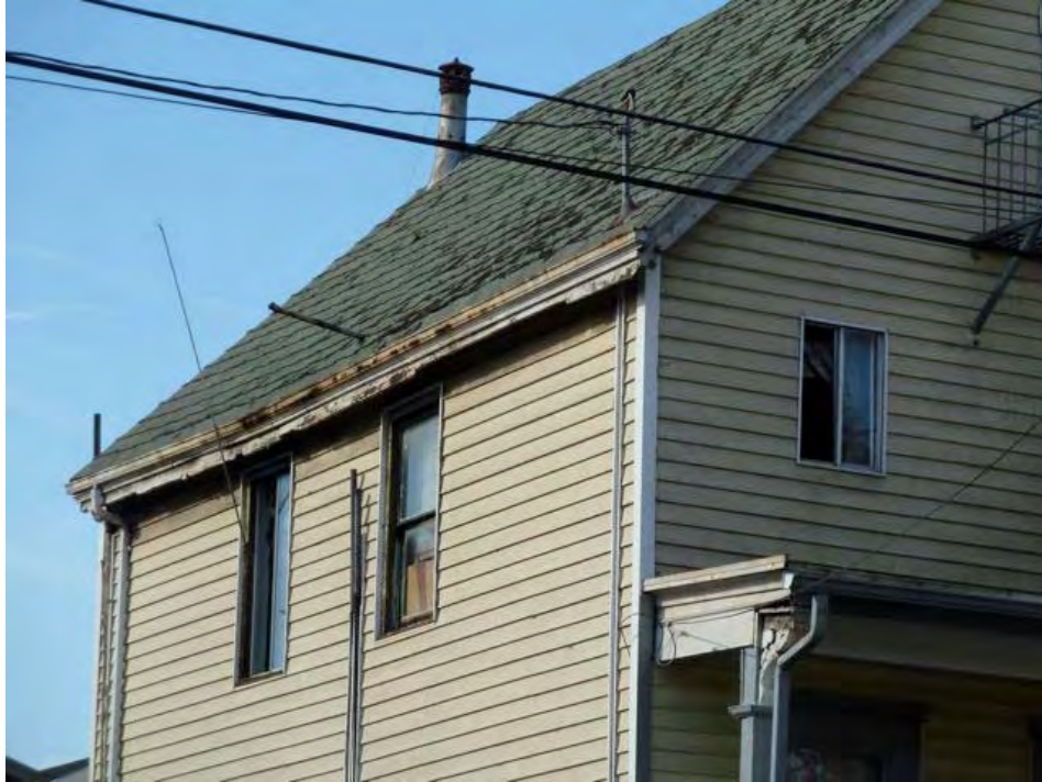
9th Street and Martin Luther King: severe roof dilapidation likely allowing moisture intrusion, mold contamination and structural wood rot.
