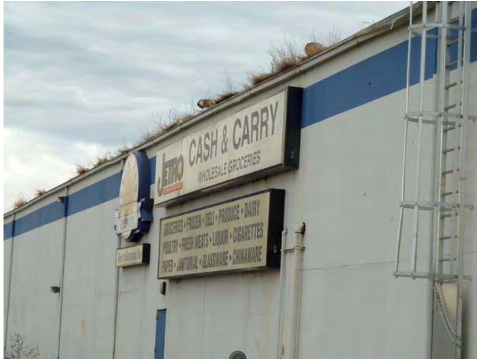
1st Street near Estuary Park: deteriorated roof and gutters likely allowing moisture intrusion, mold contamination and structural wood rot.
