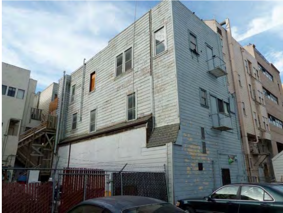
15th Street and Jefferson: serious deterioration apparently due to long-term neglect, separated siding, peeling paint, dry rot, boarded windows.
