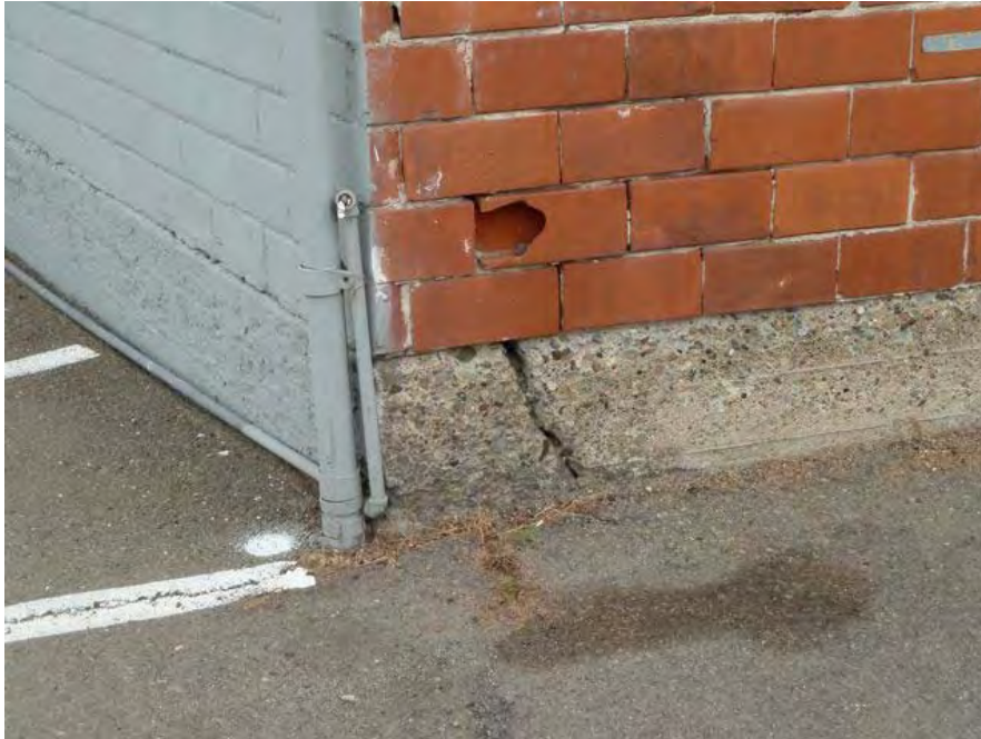
24th Street and Valley: cracked foundation.
