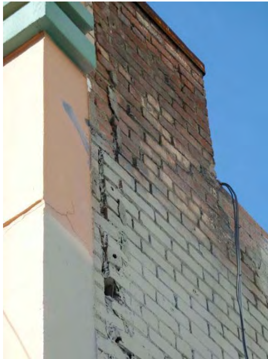
15th Street and Franklin (same building as previous photo): cracked masonry wall and separated facade potentially hazardous in event of earthquake, building vulnerable to serious damage from seismic events.
