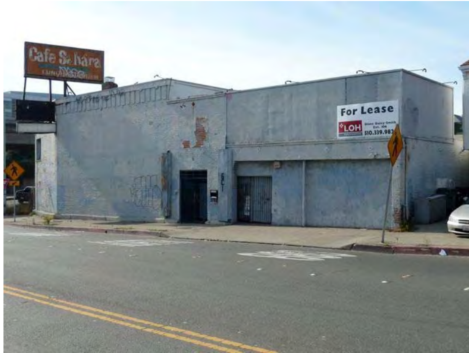
6th Street and Jackson: vacant commercial building with vandalism, partially reinforced masonry building vulnerable to serious damage from seismic events, potentially hazardous in event of earthquake.
