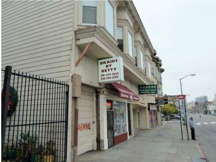
25th Street and Telegraph: structural support problems observed at building awning, deteriorated facade.
