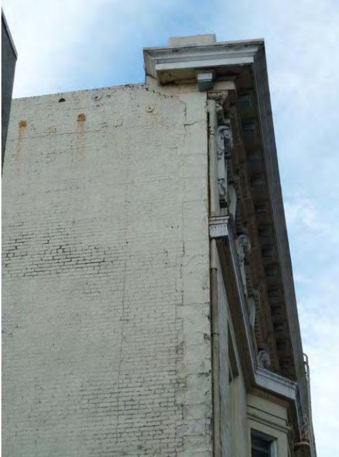
16th Street and Jefferson: partially reinforced masonry building vulnerable to serious damage from seismic events, cracked wall, separated facade from masonry wall potentially hazardous in event of earthquake.
