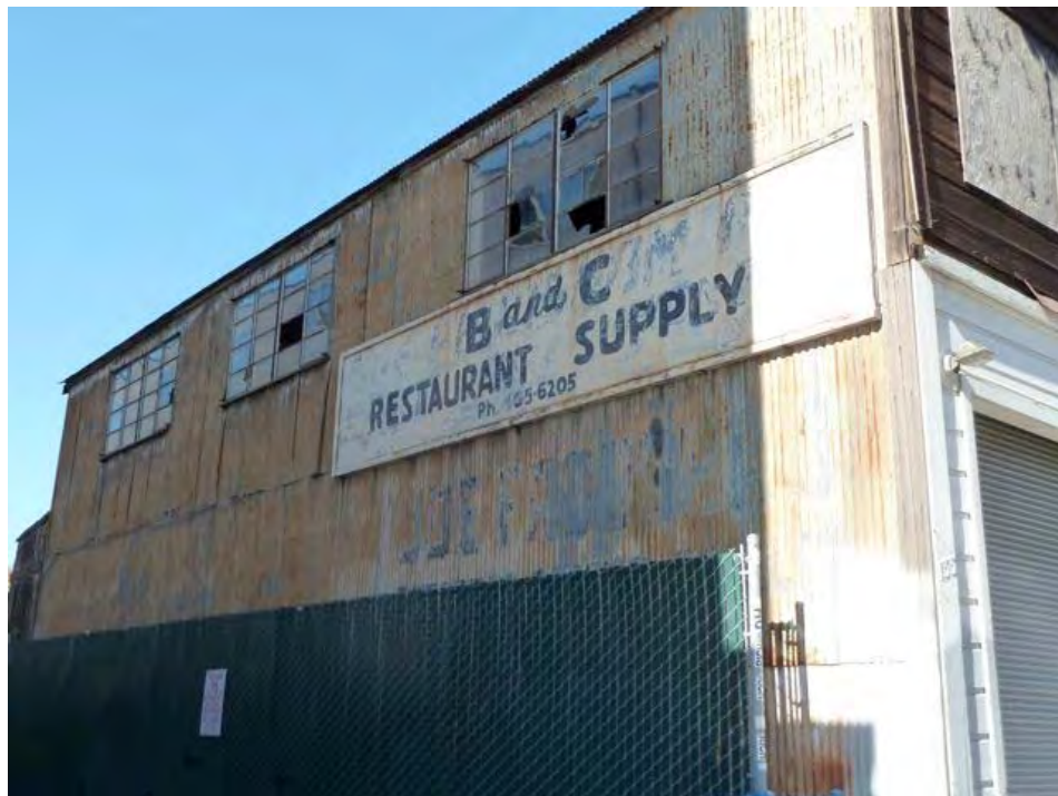
2nd Street and Franklin: broken windows, separated siding, peeling paint, and serious signage deterioration due to long-term neglect.
