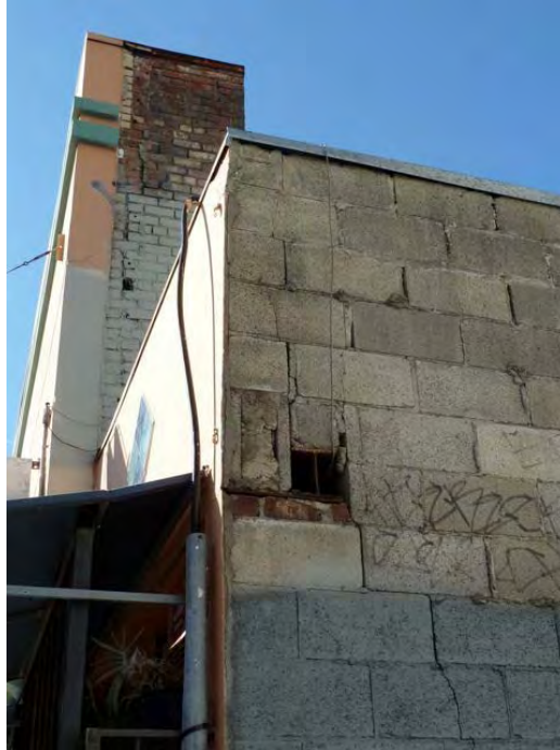
15th Street and Franklin (close up of above): deteriorated masonry wall and concrete block wall potentially hazardous in event of earthquake, building vulnerable to serious damage from seismic events.
