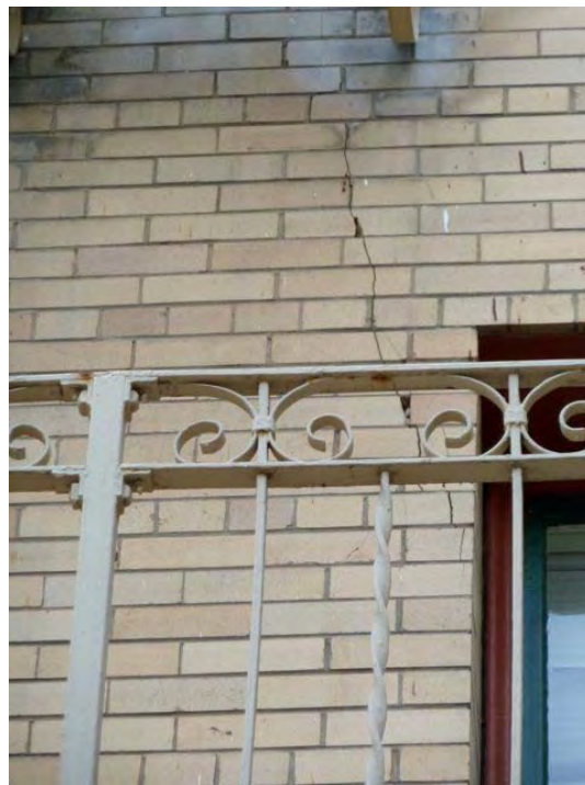
14th Street and Alice: cracked masonry wall potentially hazardous in event of earthquake, building vulnerable to serious damage in event of earthquake.
