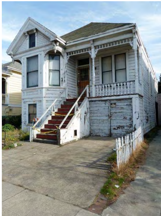
7th Street and Jackson: serious deterioration and dilapidation apparently due to long-term neglect, peeling paint, dry rot, missing and boarded windows.
