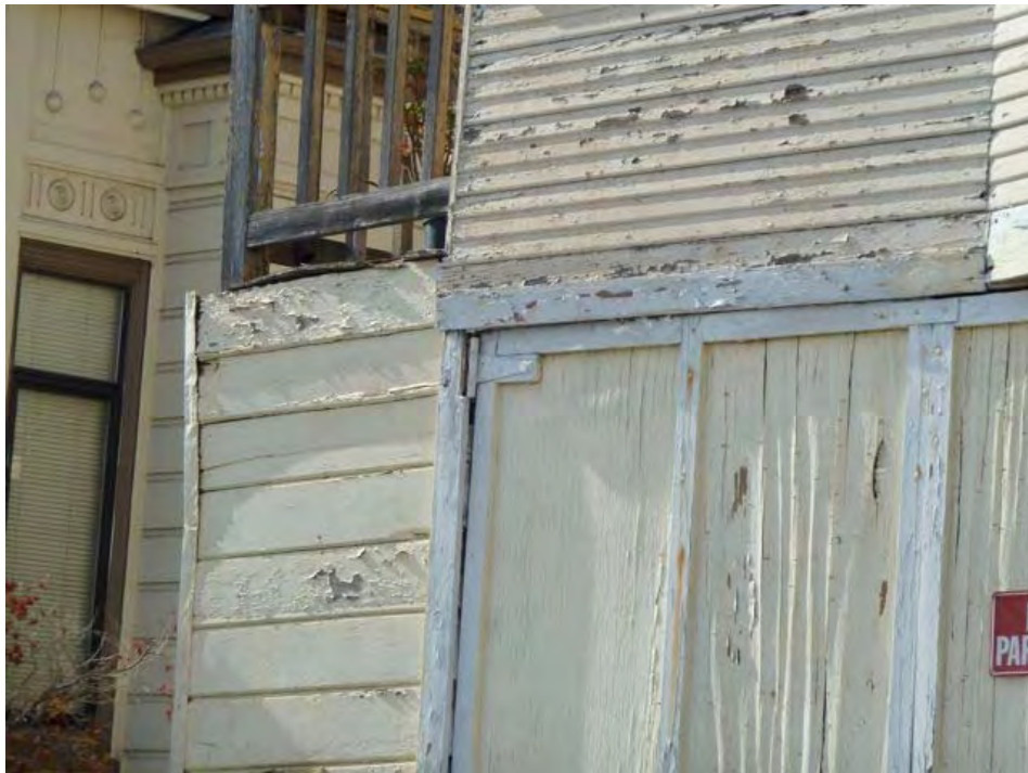
7th Street and Oak: structural alignment problems observed at porch, peeling paint, dry rot.
