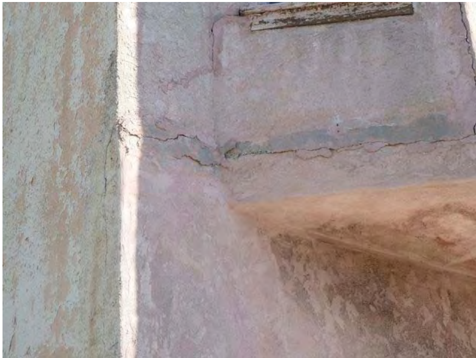
9th Street and Madison (close up of above): cracked walls, peeling paint.
