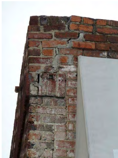
23rd Street and Valley (same building as previous photo): deteriorated and separated masonry walls at building corner potentially hazardous in event of earthquake, building vulnerable to serious damage from seismic events.
