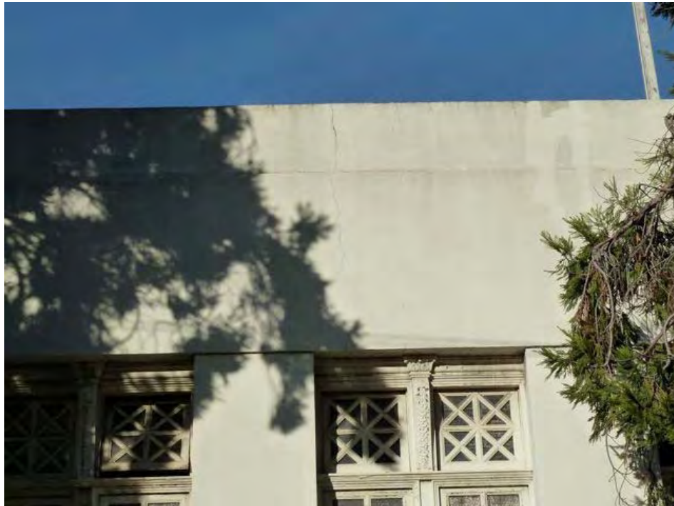
13th Street and Lakeside: cracked walls and peeling paint apparently due to long-term neglect.
