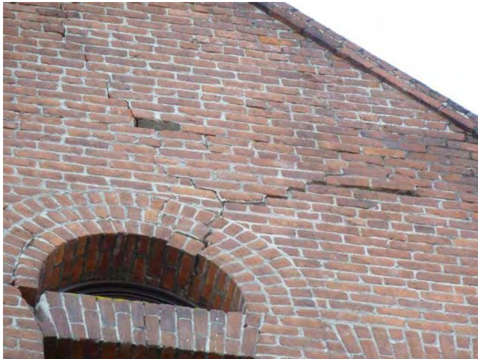
Grand and Valdez (close up of above): cracked and deteriorated masonry wall potentially hazardous in event of earthquake, building vulnerable to serious damage from seismic events.
