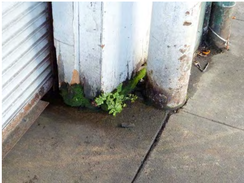
2nd Street and Broadway: deteriorated structural support.
