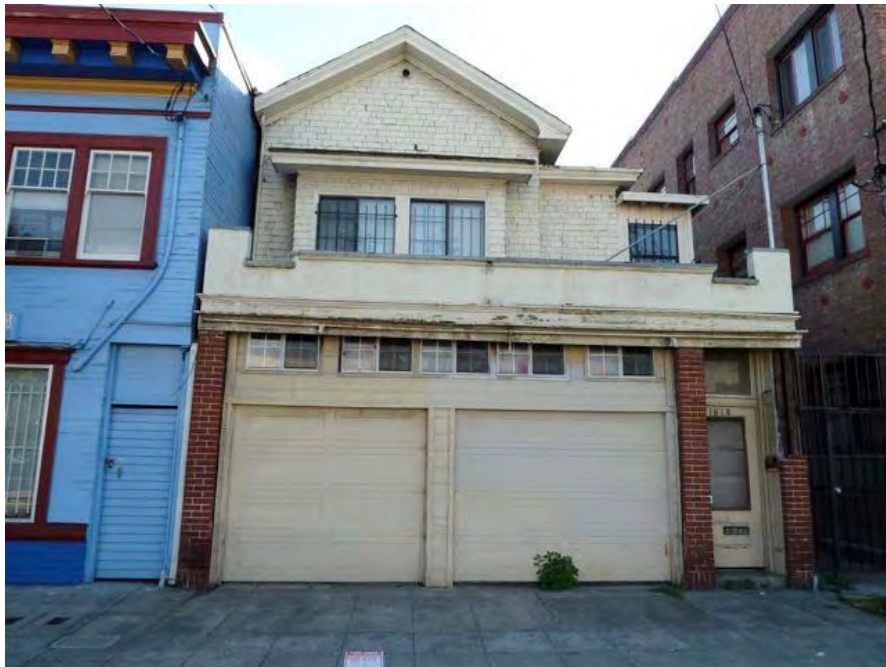
17th Street and Martin Luther King: deteriorated siding, peeling paint and dry rot apparently due to long-term neglect.
