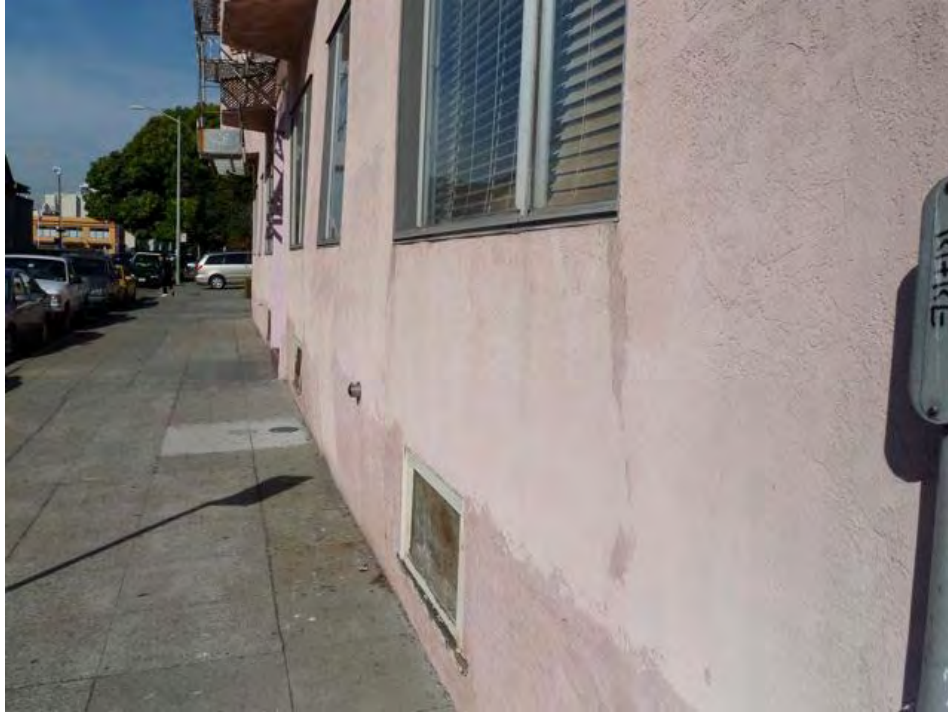
9th Street and Madison (same building as previous photo): buckling walls indicating structural alignment problems.
