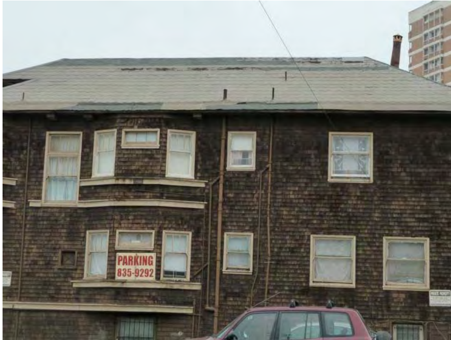
24th Street and Waverly: severe roof deterioration likely allowing moisture intrusion, mold contamination and structural wood rot.
