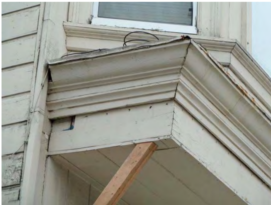
25th Street and Telegraph (close up of above): apparent separation of building awning from primary structure.
