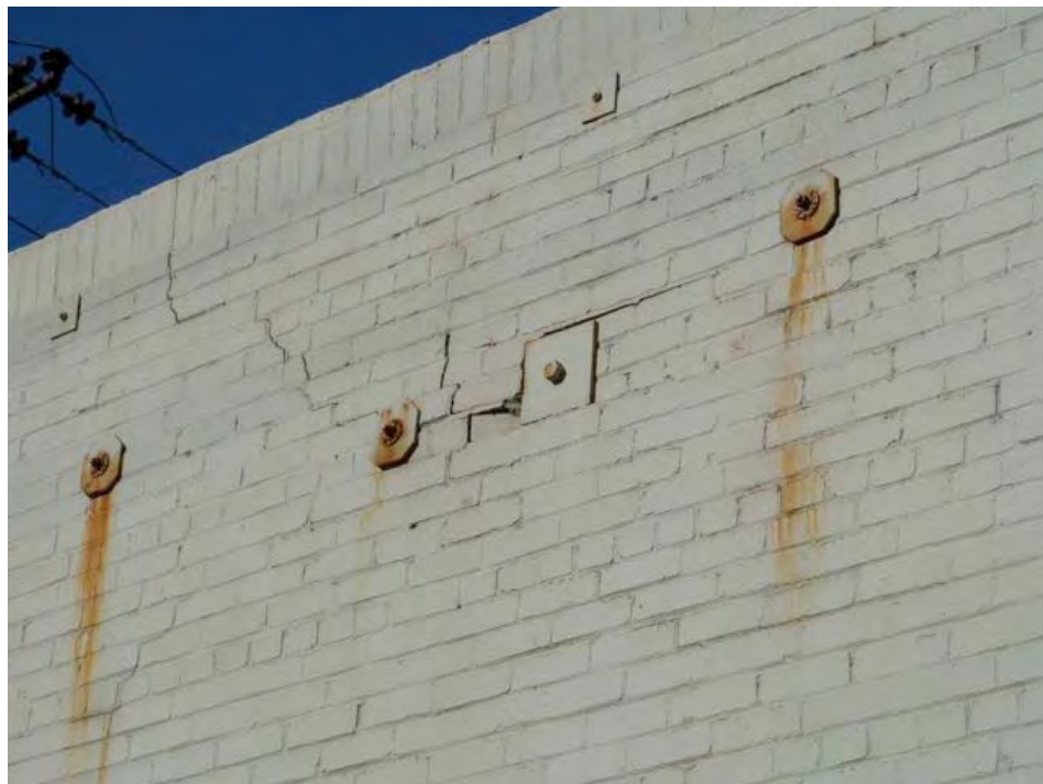
3rd Street and Castro (same building as previous photo): partially reinforced masonry building vulnerable to serious damage from seismic events, extensive cracked masonry wall potentially hazardous in event of earthquake.
