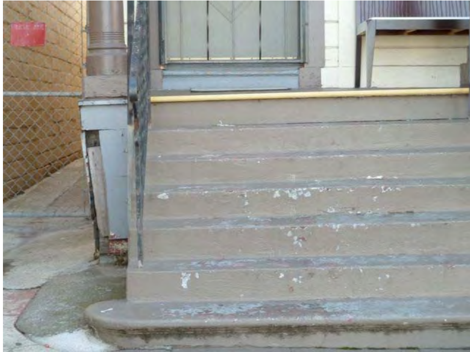
15th Street and Castro: deteriorated structural support, structural alignment problems observed at porch.
