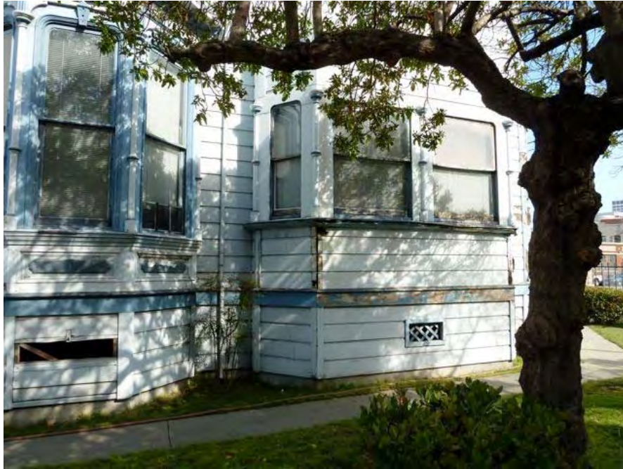
18th Street and Martin Luther King: deteriorated and missing siding, peeling paint and dry rot apparently due to long-term neglect.
