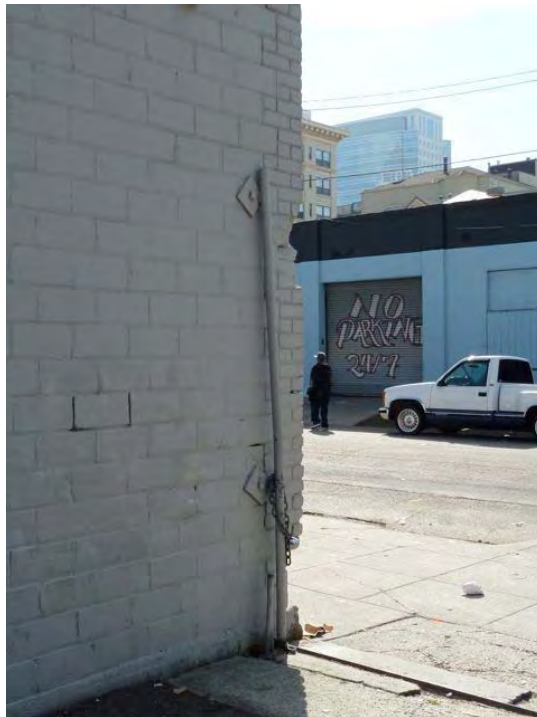
15th Street and Castro (close up of above): missing masonry along building corners potentially hazardous in event of earthquake, building vulnerable to serious damage in event of earthquake.
