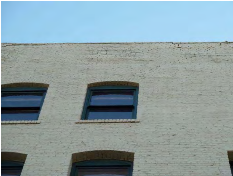
16th Street and Martin Luther King (close up of above): partially reinforced masonry building vulnerable to serious damage from seismic events, cracked and deteriorated masonry wall potentially hazardous in event of earthquake.
