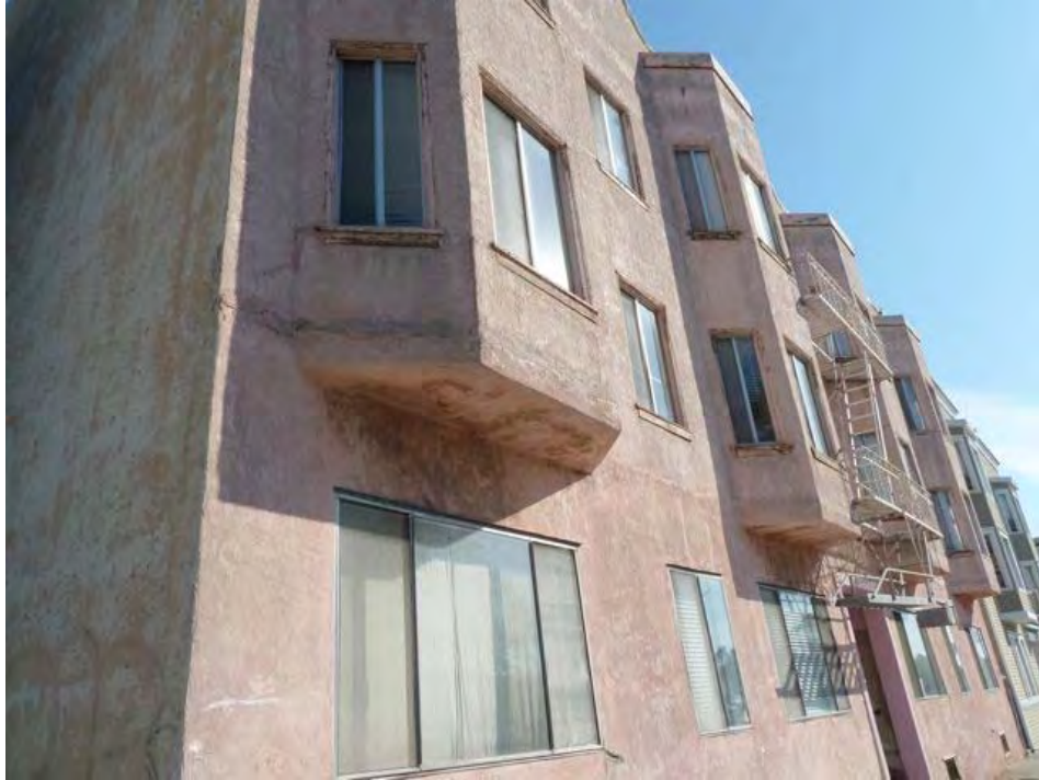
9th Street and Madison: serious deterioration apparently due to long-term neglect, peeling paint, cracked walls.
