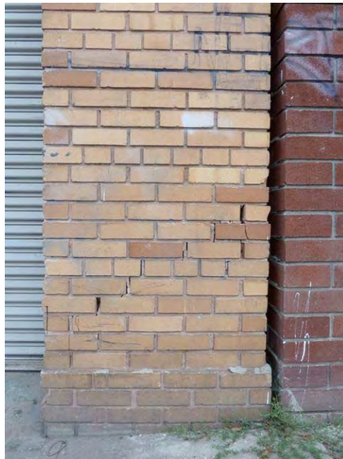
24th Street and Waverly (close up of above): cracked and deteriorated masonry wall potentially hazardous in event of earthquake, building vulnerable to serious damage in event of earthquake.
