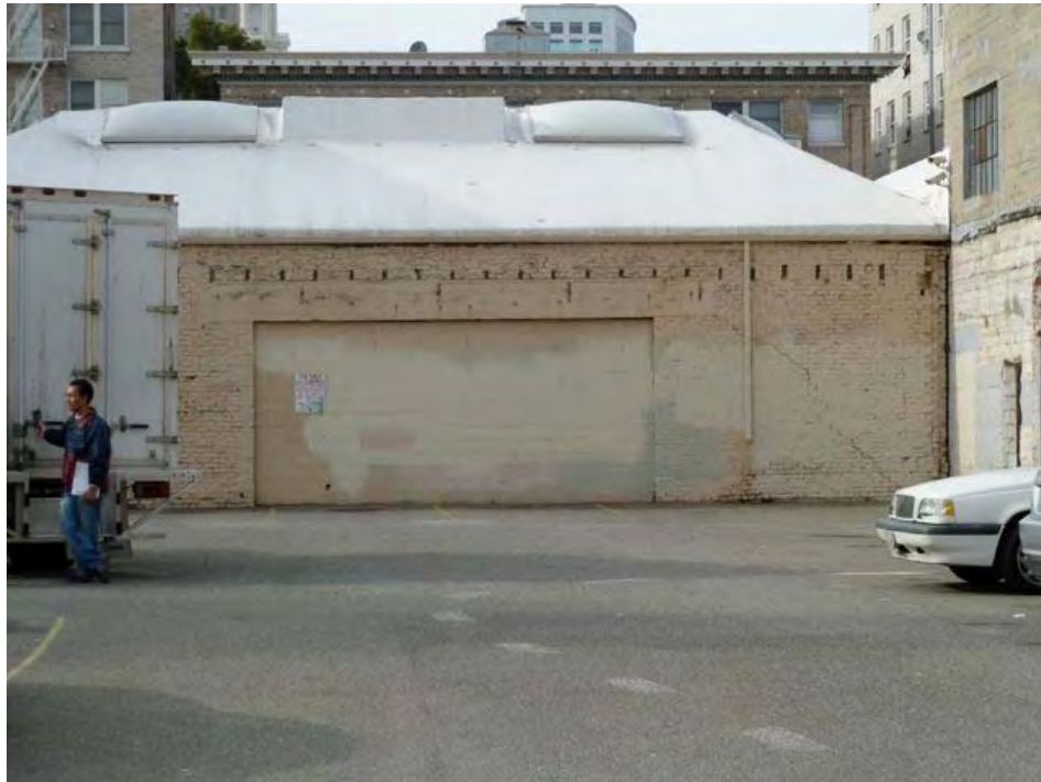
14th Street and Alice: unreinforced masonry building vulnerable to serious damage from seismic events, cracked and deteriorated masonry wall potentially hazardous in event of earthquake.
