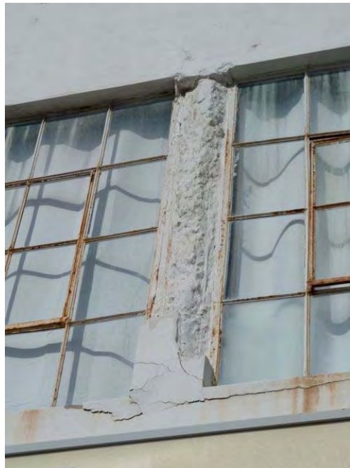
25th Street and Telegraph: deteriorated and cracked wall near windows likely causing water intrusion.
