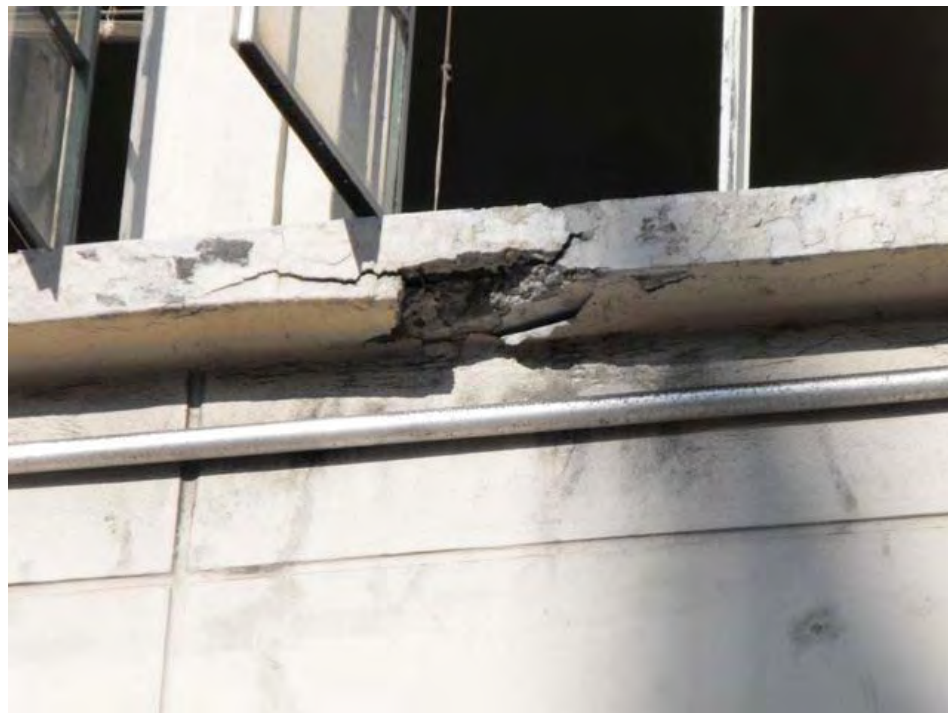
7th Street and Webster (close up of above): crumbled and deteriorated facade, apparently due to long-term neglect.
