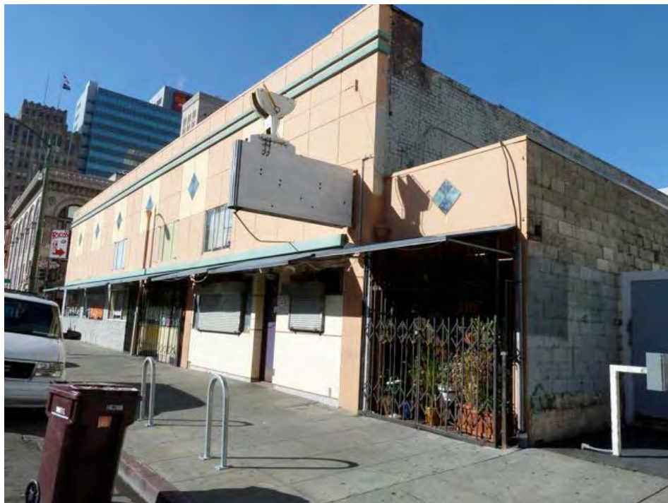
15th Street and Franklin: partially reinforced masonry building and unreinforced concrete block building vulnerable to serious damage from seismic events, deteriorated facade, deteriorated masonry potentially hazardous in event of earthquake.
