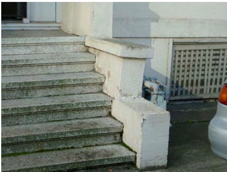
10th Street and Jefferson: structural alignment problems observed in stairs, peeling paint.
