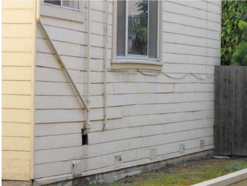
017th Street and Alice: structural alignment problems as observed in siding.
