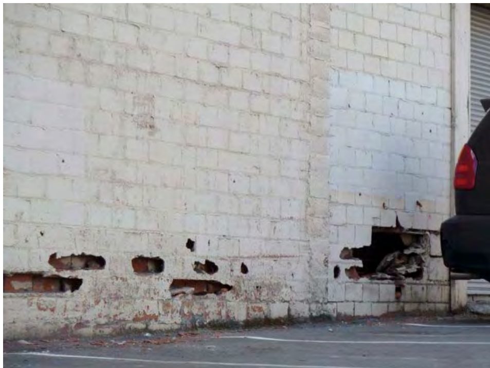
Grand and Valdez (close up of above): severely deteriorated masonry wall potentially hazardous in event of earthquake, building vulnerable to serious damage from seismic events.
