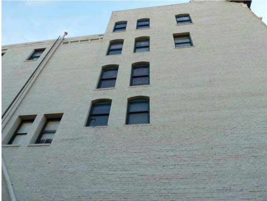
16th Street and Martin Luther King: partially reinforced masonry building vulnerable to serious damage from seismic events, building potentially hazardous in event of earthquake.
