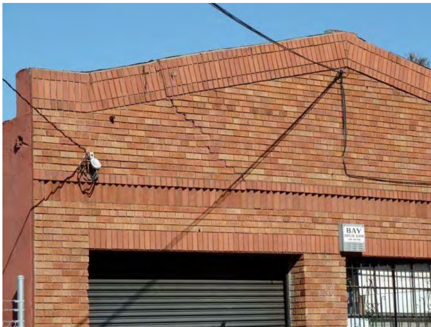
25th Street and Broadway: unreinforced masonry building vulnerable to serious damage from seismic events, cracked wall potentially hazardous in event of earthquake.
