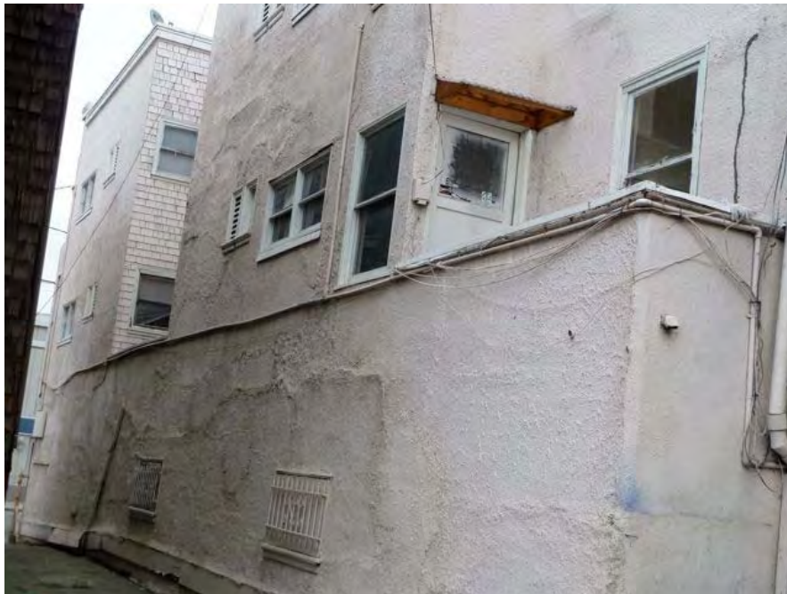
24th Street and Waverly: apparent water intrusion in building wall likely allowing mold contamination and structural wood rot.
