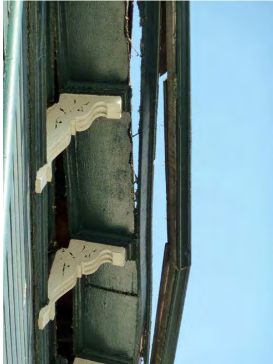
18th Street and Castro: severe eave separation likely allowing moisture intrusion, mold contamination and structural wood rot, eave deterioration.
