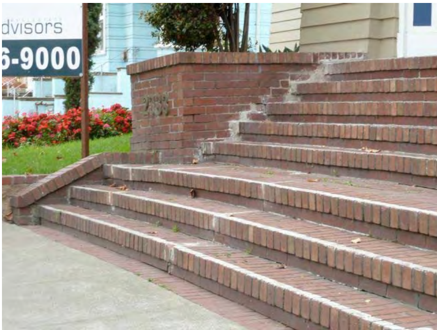
23rd Street and Harrison: cracked and deteriorated masonry stairway.
