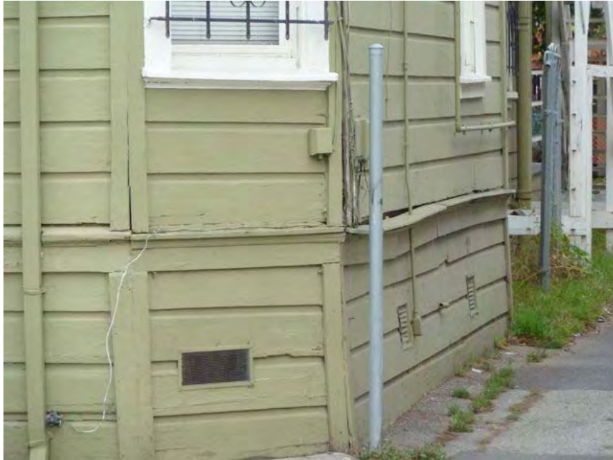
23rd Street and Valley: structural alignment problems observed in building siding, deteriorated siding, dry rot.
