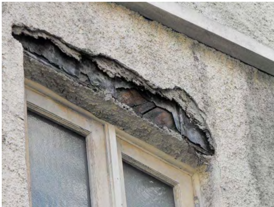
15th Street and Jackson (same building as previous photo): deteriorated siding likely allowing moisture intrusion, mold contamination and structural wood rot.
