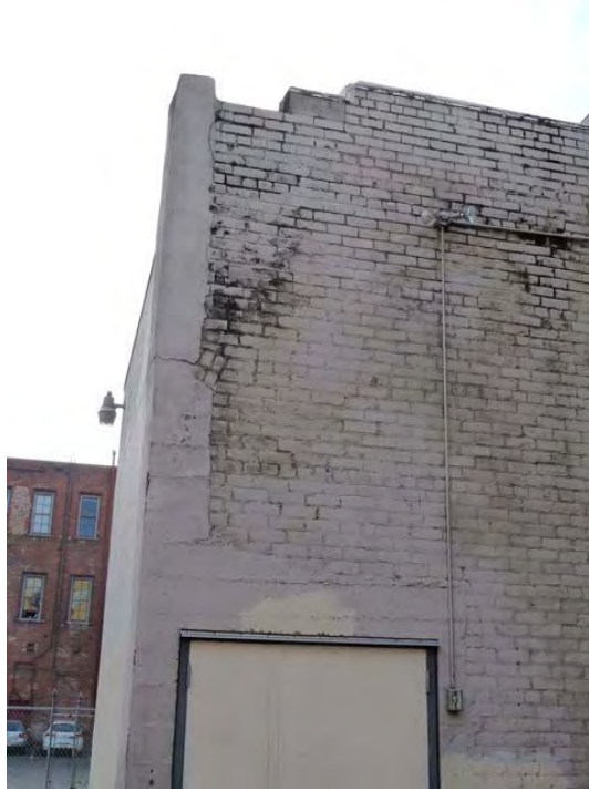
9th Street and Clay: unreinforced masonry building vulnerable to serious damage from seismic events, cracked and deteriorated wall potentially hazardous in event of earthquake, peeling paint.
