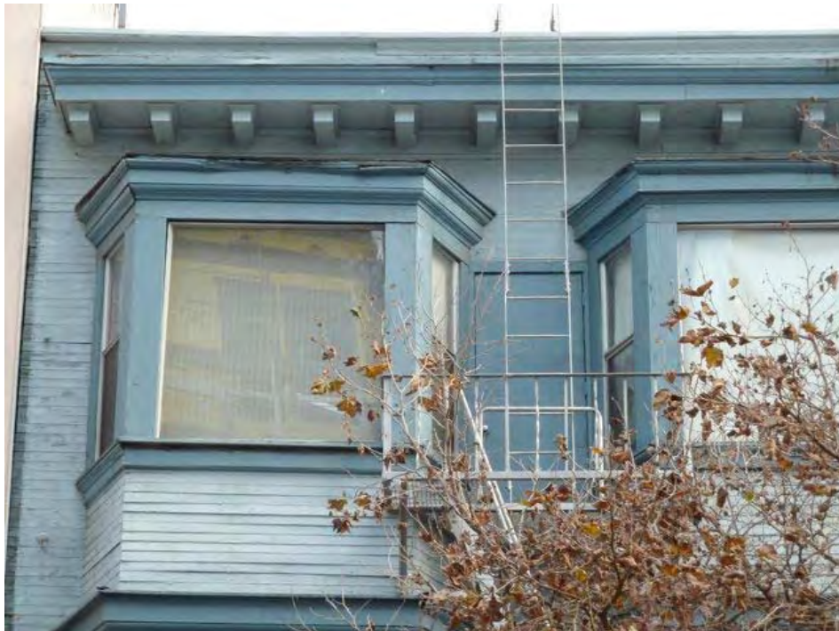
15th Street and Jefferson (close up of above): peeling paint, dry rot, deteriorated siding.
