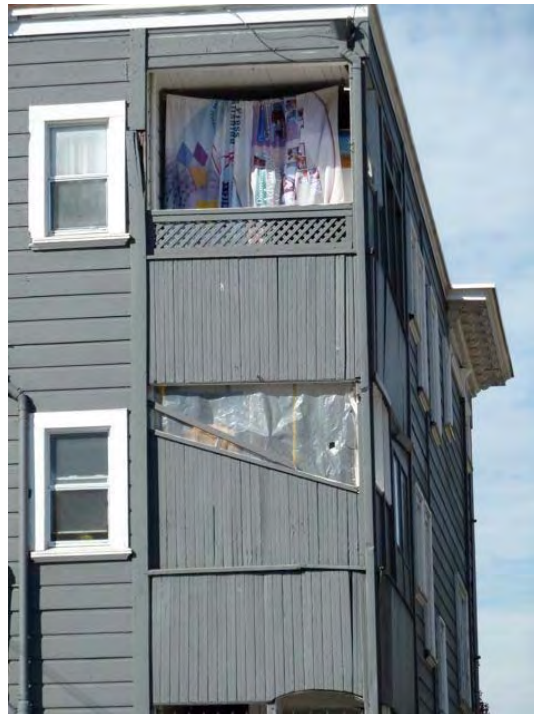
15th Street and Castro: structural alignment problems observed at balcony, missing windows, peeling paint.
