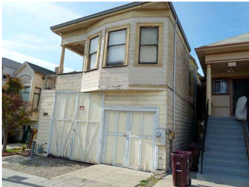
7th Street and Oak: serious deterioration apparently due to long-term neglect, peeling paint, dry rot.
