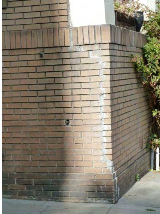
17th Street and Alice (same building as previous photo): cracked masonry at building corner potentially hazardous in event of earthquake, building vulnerable to serious damage in event of earthquake.
