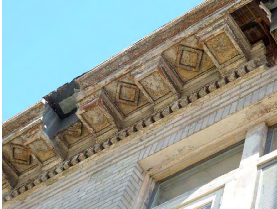
19th Street and Telegraph: apparent long-term neglect, peeling paint, deteriorating roof and eaves likely allowing moisture intrusion and mold contamination.
