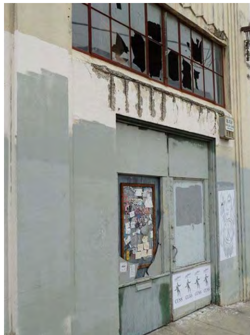
24th Street and Valley (same building as previous photo): broken and boarded windows, cracked wall, deteriorated concrete facade with exposed rebar.
