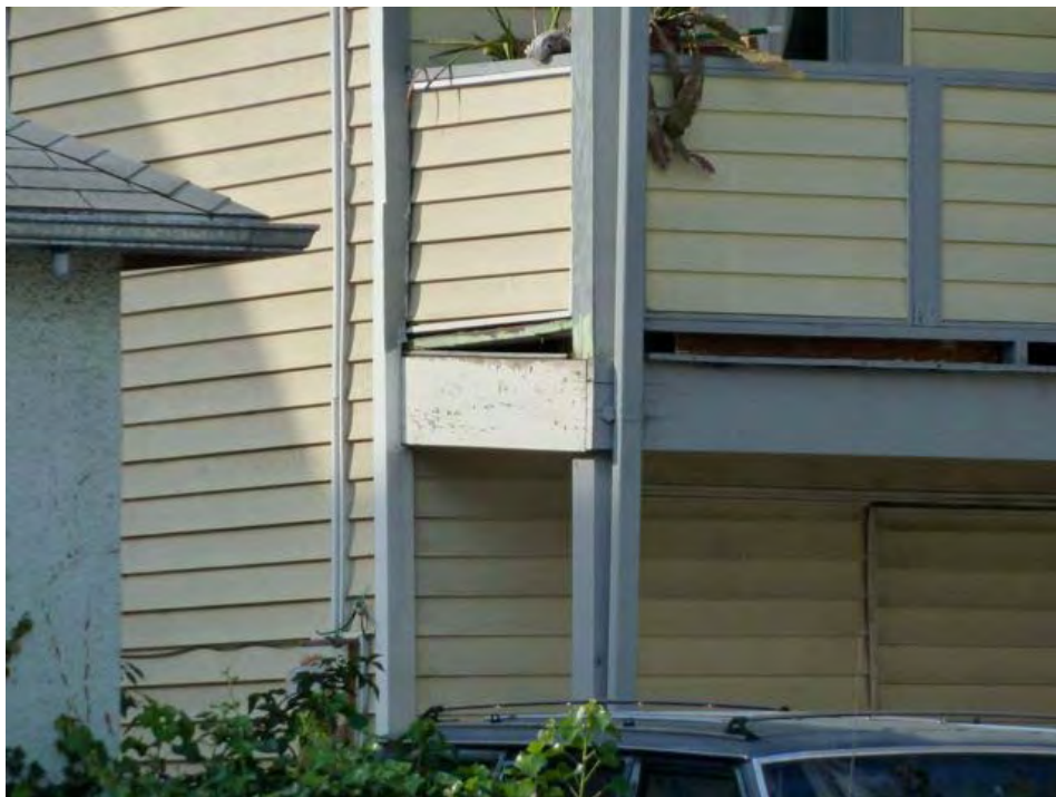
9th Street and Martin Luther King (same building as previous photo): structural alignment problems observed at porch.
