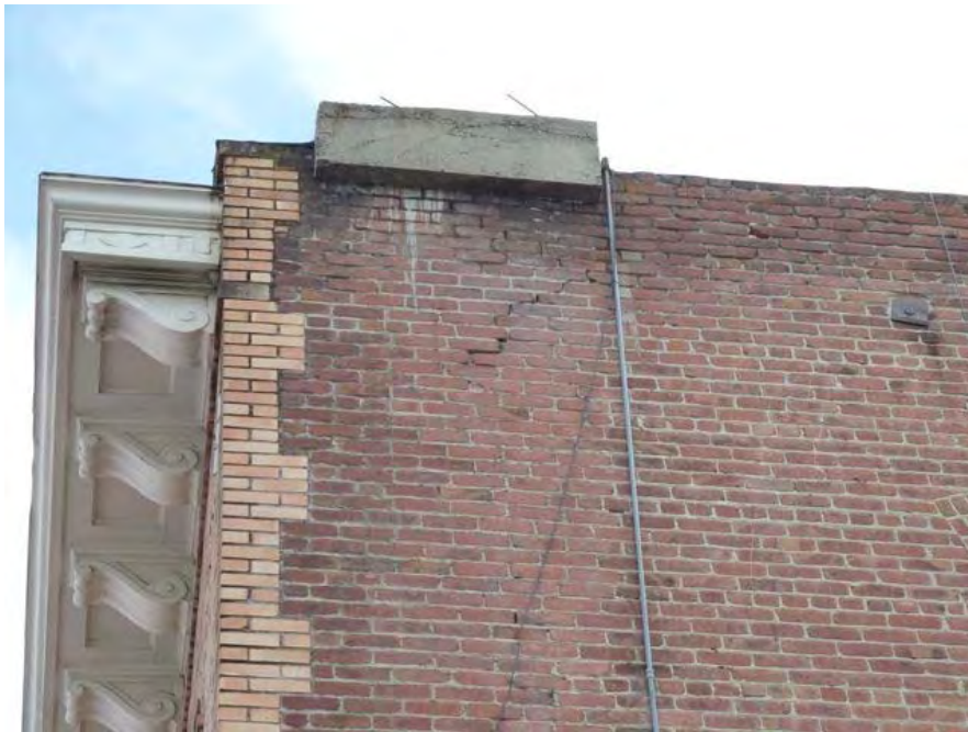
26th Street and Telegraph: partially reinforced masonry building vulnerable to serious damage from seismic events, cracked masonry wall potentially hazardous in event of earthquake.
