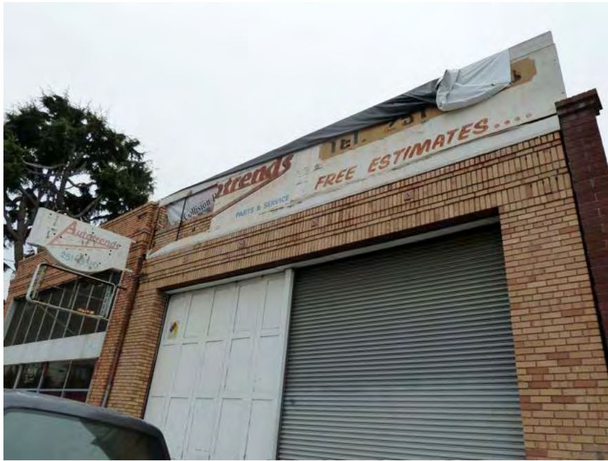
24th Street and Waverly: unreinforced masonry building vulnerable to serious damage from seismic events, building potentially hazardous in event of earthquake, deteriorated facade.
