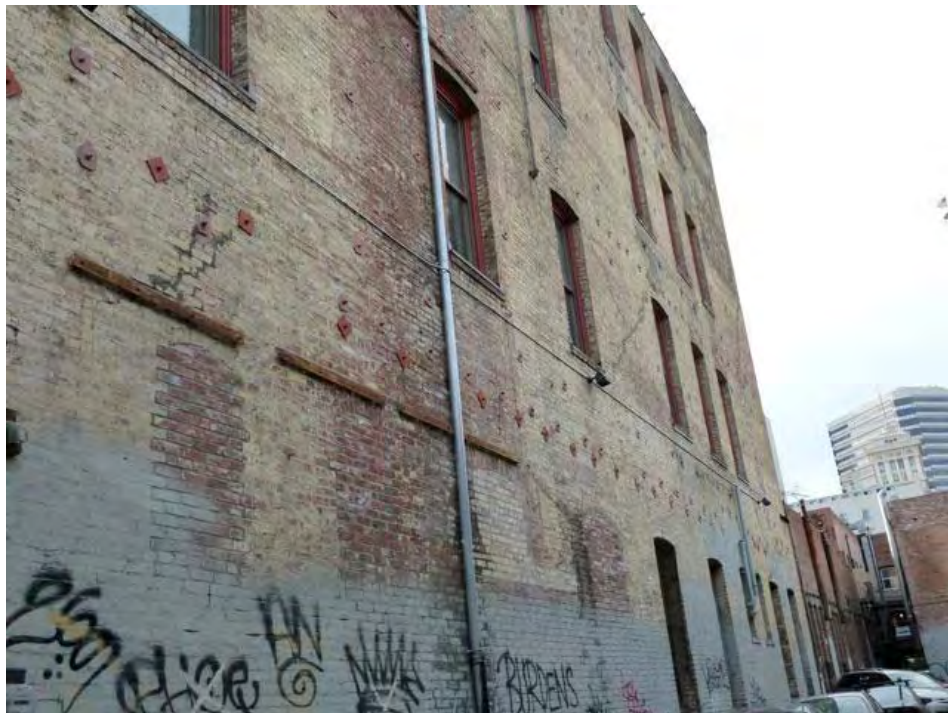
12th Street and Harrison: partially reinforced masonry building vulnerable to serious damage from seismic events, cracked masonry wall potentially hazardous in event of earthquake, graffiti.
