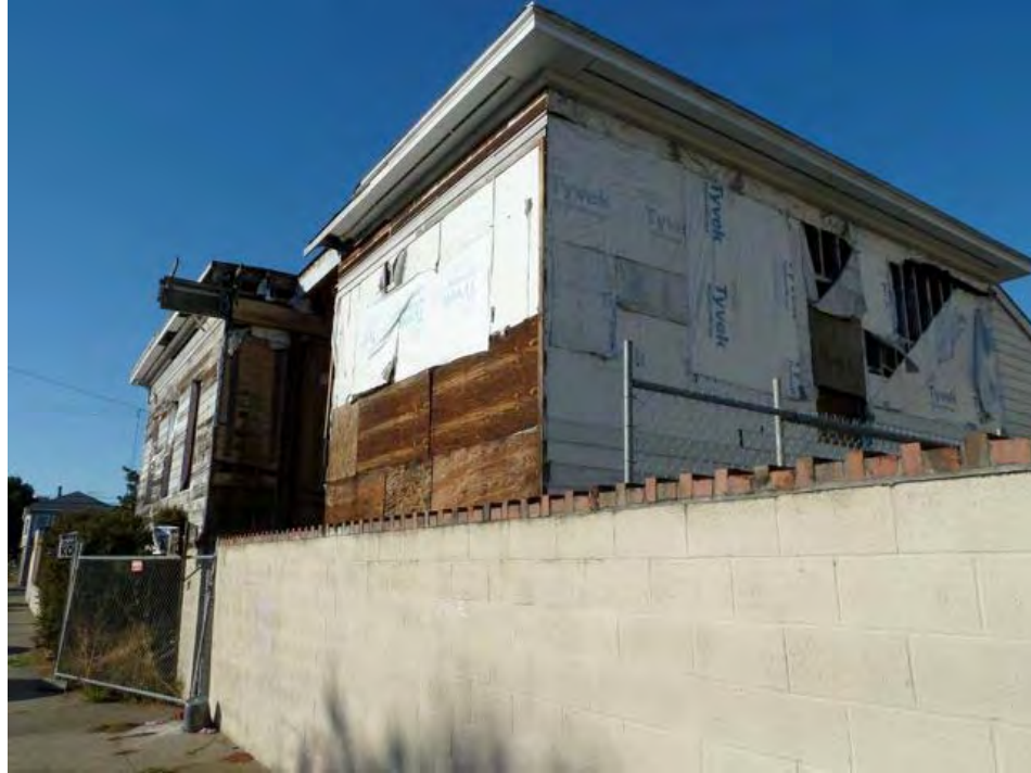
7th Street and Martin Luther King: abandoned building with substandard siding and wall materials, deteriorated siding, missing and boarded windows, peeling paint, dry rot.
