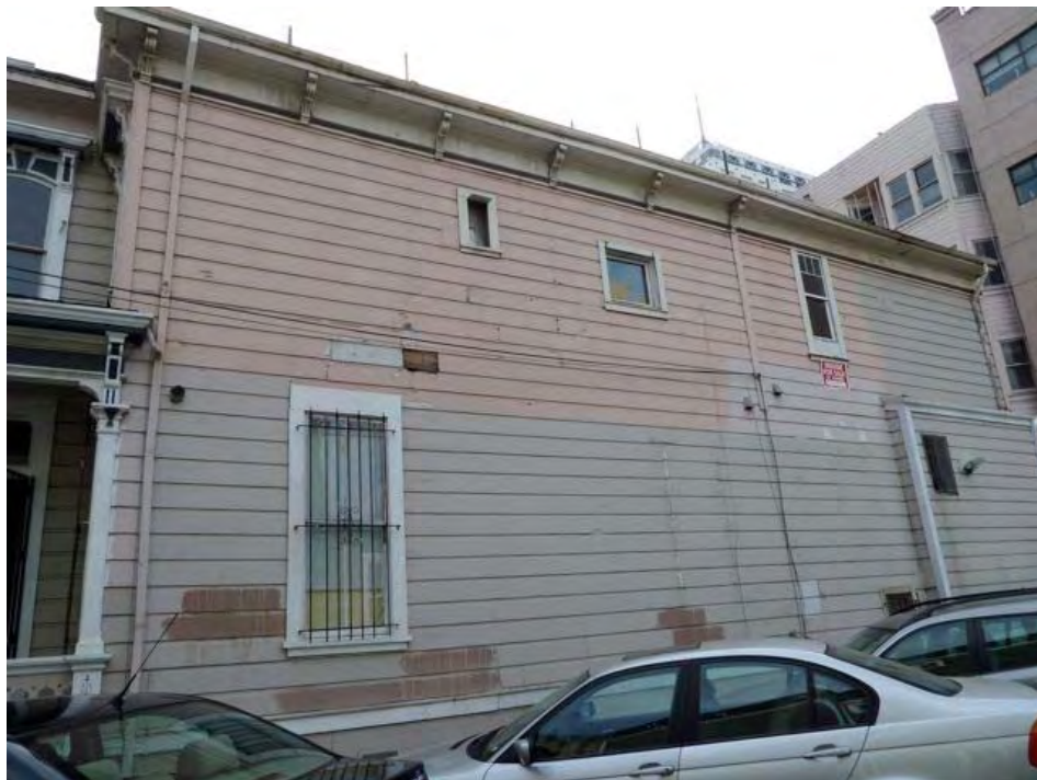
15th Street and Jefferson: deteriorated siding, peeling paint, boarded windows, and cracked wall apparently due to long-term neglect.
