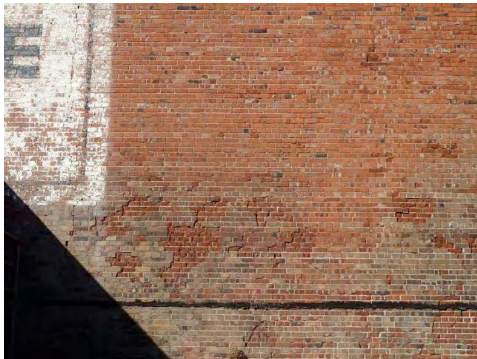
2nd Street and Clay: cracked and deteriorated masonry wall potentially hazardous in event of earthquake, building vulnerable to serious damage from seismic events.
