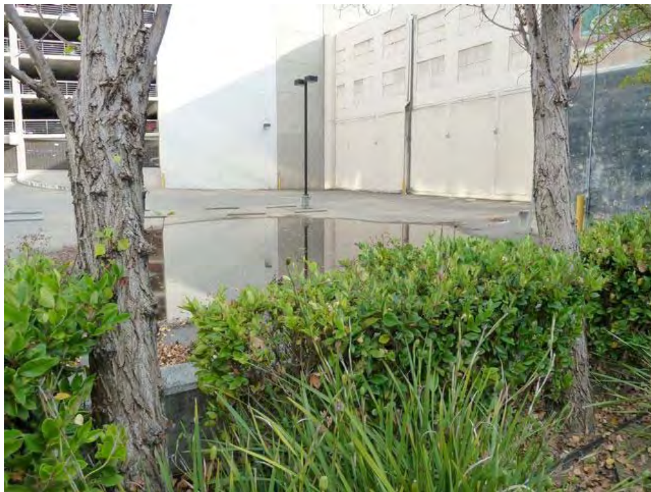
19th Street and Broadway: standing water apparently due to inadequate drainage.
