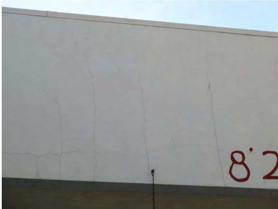
14th Street and Jackson: multiple wall cracks suggest structural issue.
