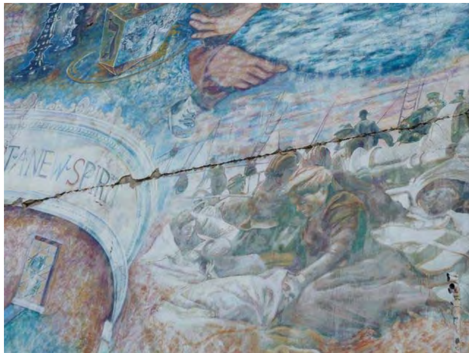
14th Street and Franklin (close up of above): horizontal crack across building.
