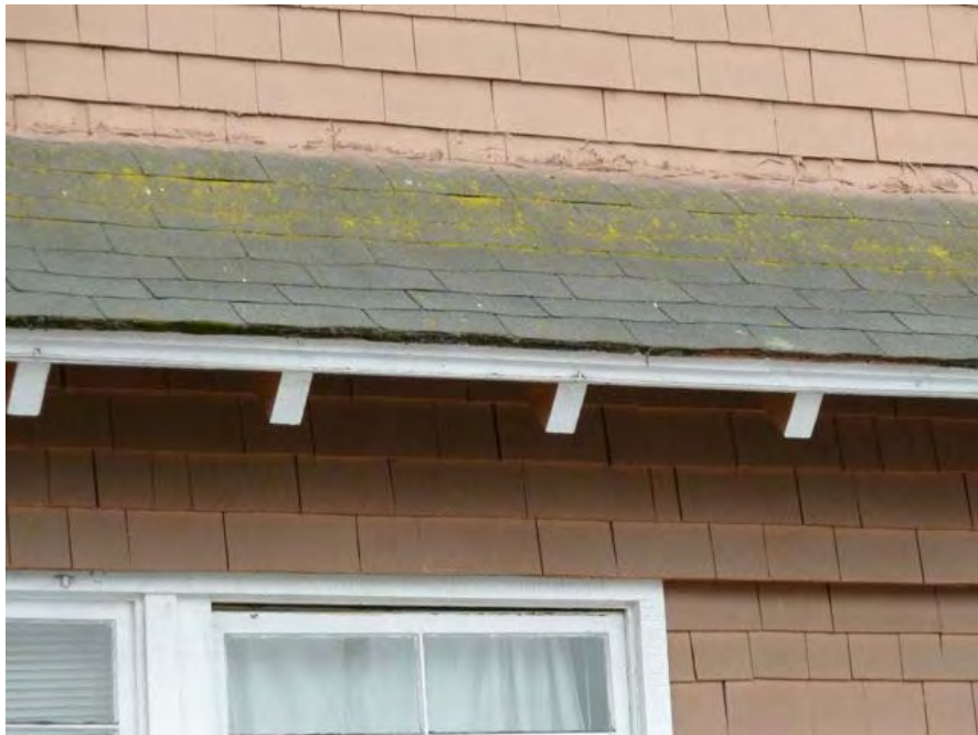
24th Street and Waverly (close up of above): deteriorated roof likely allowing moisture intrusion, mold contamination and structural wood rot.
