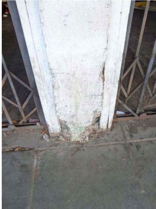
2nd Street and Franklin: deteriorated structural support.
