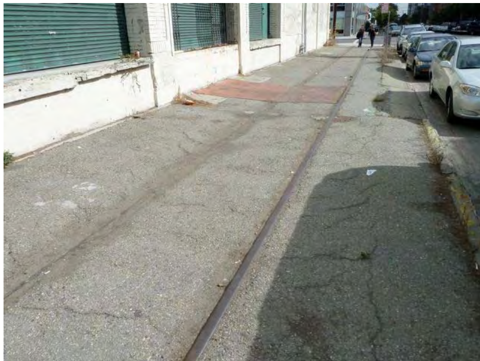
4th Street and Harrison: deteriorated and inadequate sidewalk, abandoned and defunct rail lines.
