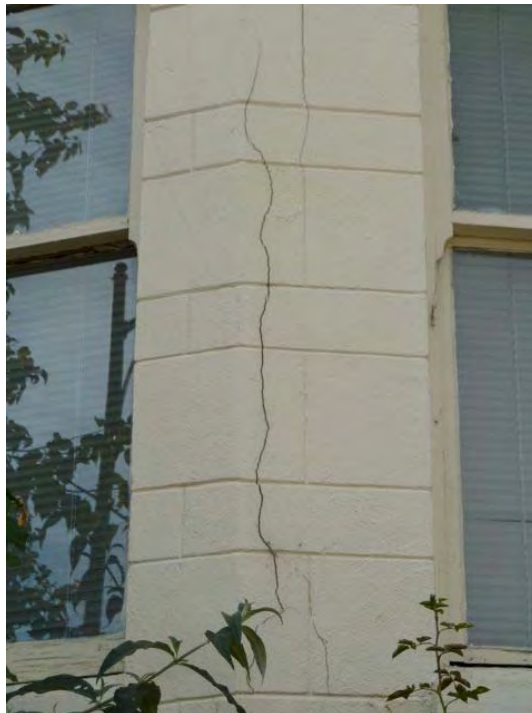
17th Street and Alice (same building as previous photo): cracked wall near windows.
