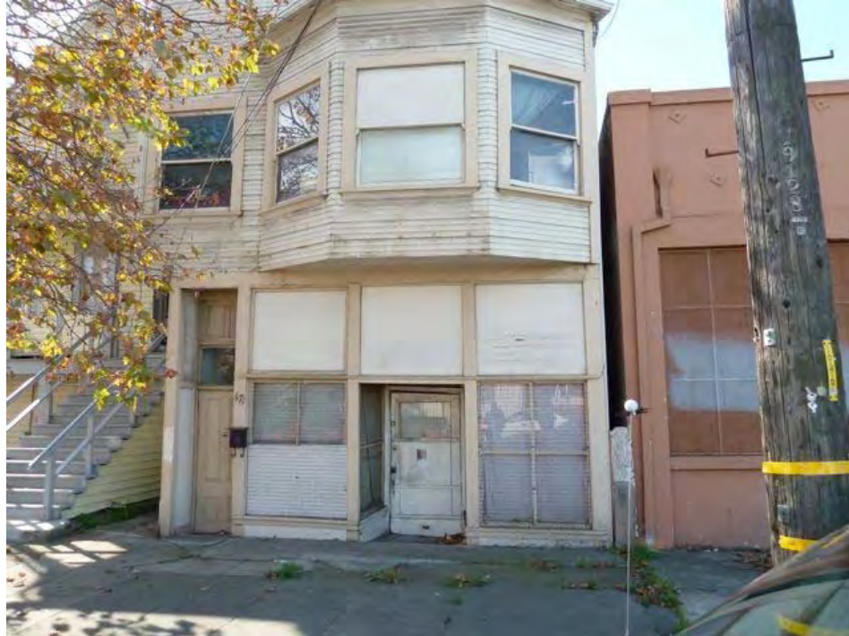
9th Street and Castro: deteriorated siding, peeling paint and boarded windows apparently due to long-term neglect.
