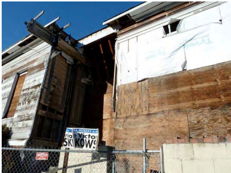
7th Street and Martin Luther King (close up of above): serious deterioration and dilapidation apparently due to long-term neglect, deteriorated siding, wood rot, peeling paint.
