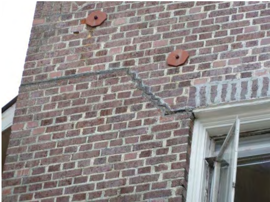
Bay Place and Access Road: cracked masonry wall potentially hazardous in event of earthquake, building vulnerable to serious damage in event of earthquake.
