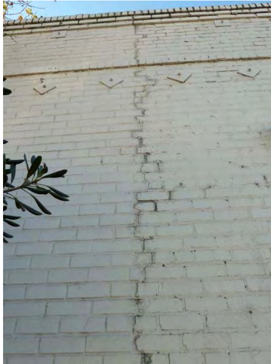
3rd Street and Jefferson: partially reinforced building vulnerable to serious damage from seismic events, severe cracked masonry potentially hazardous in event of earthquake.
