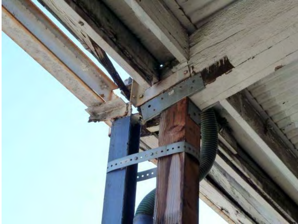
2nd Street and Franklin (same building as previous photo): deteriorated and separated structural support.
