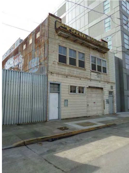
5th Street and Jackson: peeling paint and deteriorated and separated siding apparently due to long-term neglect.
