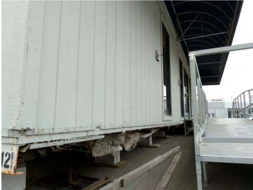
27th Street and Broadway: apparent long-term neglect evidenced by deterioration of building floor.
