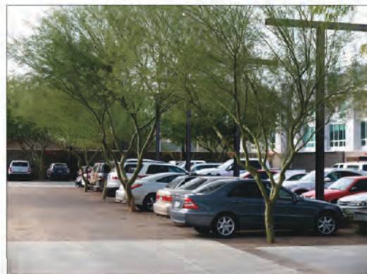
Figure 3.11.i: This multi-family project utilizes gravel driveways and concrete slabs in its adjacent parking lot that allow stormwater to infiltrate.
