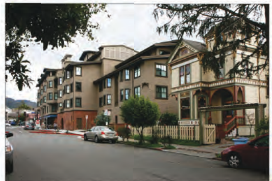
Figures 4.2.b and 4.2.c: The new residential building (top) is scaled to match the surrounding single-family homes, and is composed of varied scales and articulation of height and massing; another residential building (bottom) transitions in height and setback to match the existing single-family home next door.
