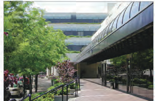
Figure 4.5.c: The smoked glass frontage of the building's street level facade provides privacy for interior offices, but does little to create a visibly active frontage along the sidewalk. It essentially creates a blank wall condition.
