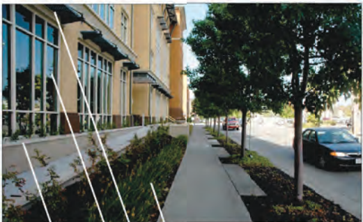
landscaped setback sun shades on windows high transparency raised interior floor
