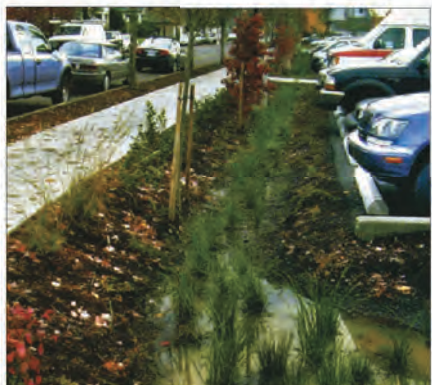
► 3.11.h: This vegetated swale collects runoff from the adjacent parking lot and sidewalk and slows and treats the stormwater prior to release into the storm drain system.
