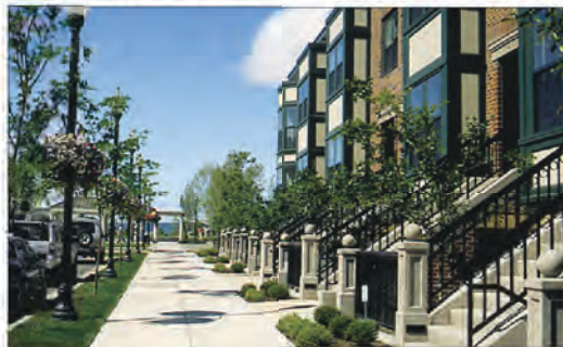
Figure 4.4.c: Open railings on these entry stairs preserve the sight line along the building setback creating an open, inviting transition by creating a continuous semi-public space.
