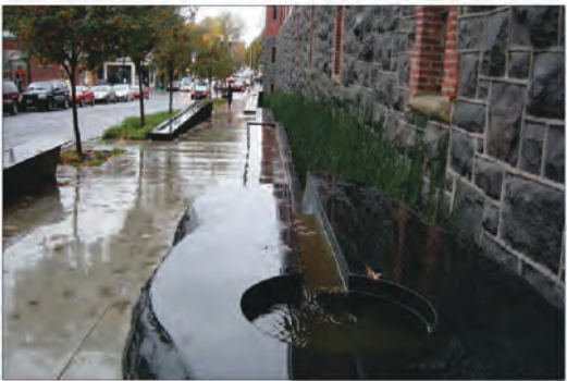
► Figure 3.11.f: This stormwater channel serves a dual purpose of containing runoff and providing visual interest at the street level.
