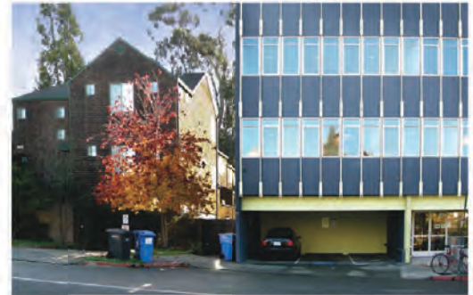
Figure 4.2.a: The siting, massing, articulation and height of the office building on the right disregards the existing character of the adjacent residential neighborhood.
