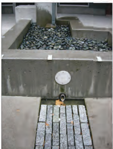
► Figure 3.11.b: This facility gathers rooftop runoff and funnels it to a ground level water feature before it reaches the storm drain system, slowing and filtering the flow.
