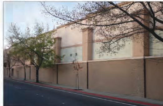
Figure 4.6.a: The articulation on this long stretch of blank wall is too repetitive in form, color and material to create an engaging façade along the sidewalk.
