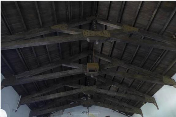
Figure 32: Scissor trusses, 2013.
