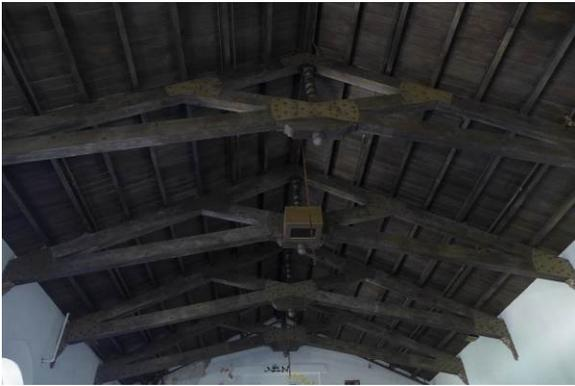
Figure 32: Scissor trusses, 2013.
