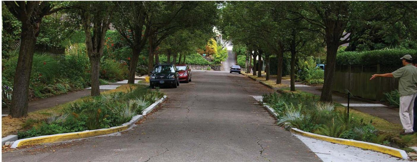
Typical Infiltration Bulb-out / Flow-through Planter / Rain Garden
