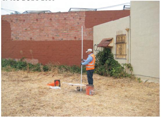
Photograph 18: Driller Removing Temporary PVC Casings from Boring B-01.
