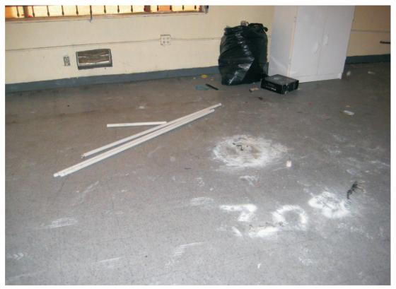
Photograph 21: Driller Removed Temporary PVC Casings from Boring B-02 prior to Grouting.
