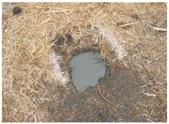
Photograph 23: Grouted Boring B-01 to Ground Surface.
