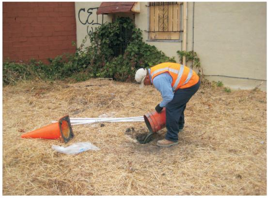
Photograph 19: Driller Grouting Boring B-01 with Neat Cement.
