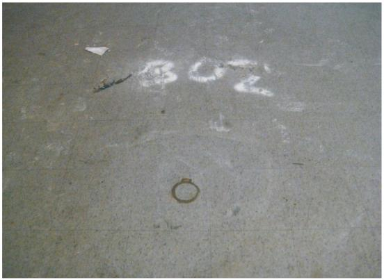
Photograph 24: Grouted Boring B-02 to Ground Surface.
