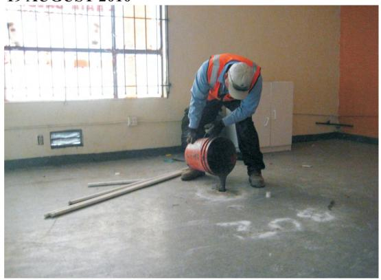
Photograph 22: Driller Grouting Boring B-02 with Neat Cement.
