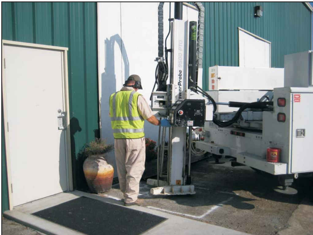
Photograph 22: TEG installing shallow probe at SG-03.
