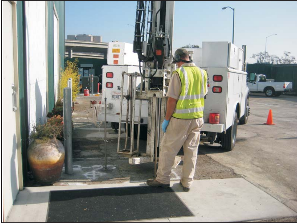
Photograph 23: TEG installing deep probe at SG-03.
