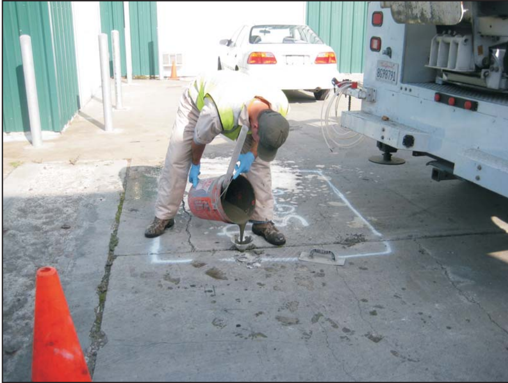
Photograph 17: TEG grouting of shallow boring at SG-05.
