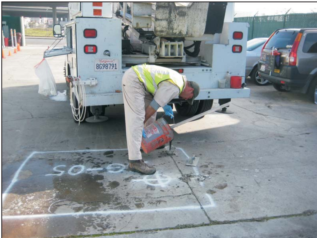
Photograph 16: TEG grouting of deep boring at SG-05.
