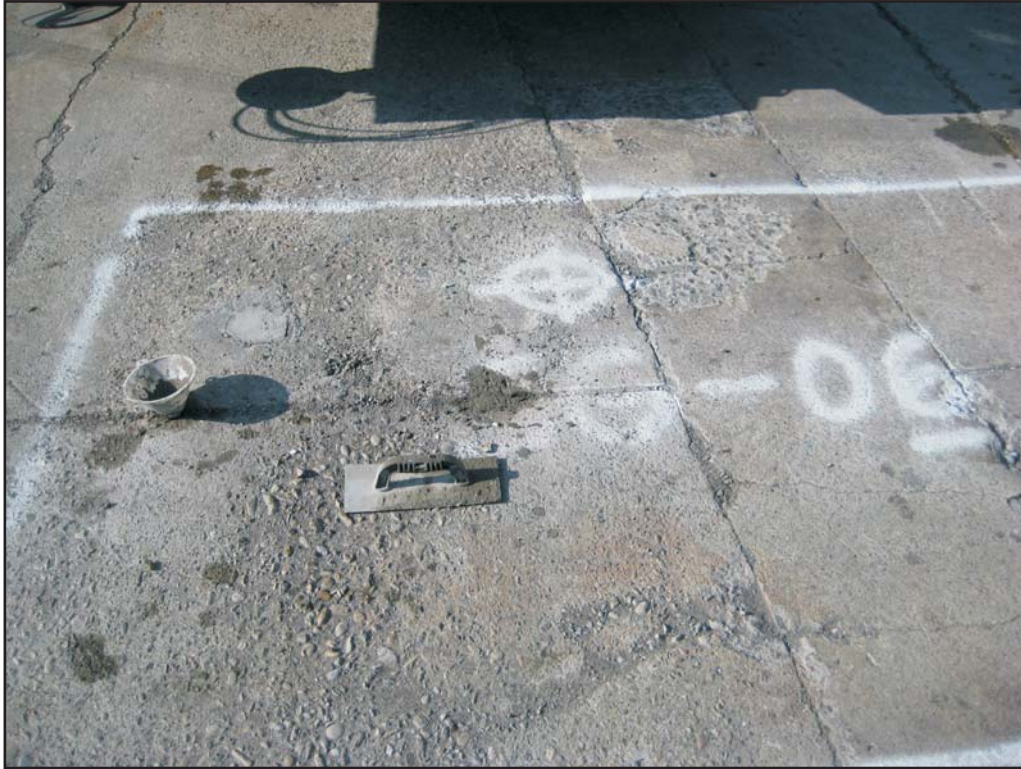
Photograph 21: Abandonment of boreholes at SG-06.
