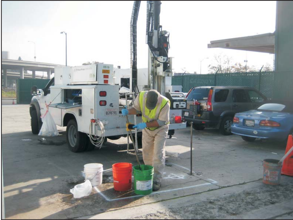
Photograph 15: TEG decontamination of probes removed from SG-05.
