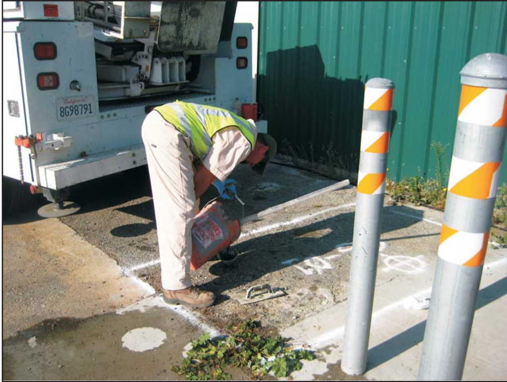
Photograph 25: TEG abandoning of boreholes at SG-01.
