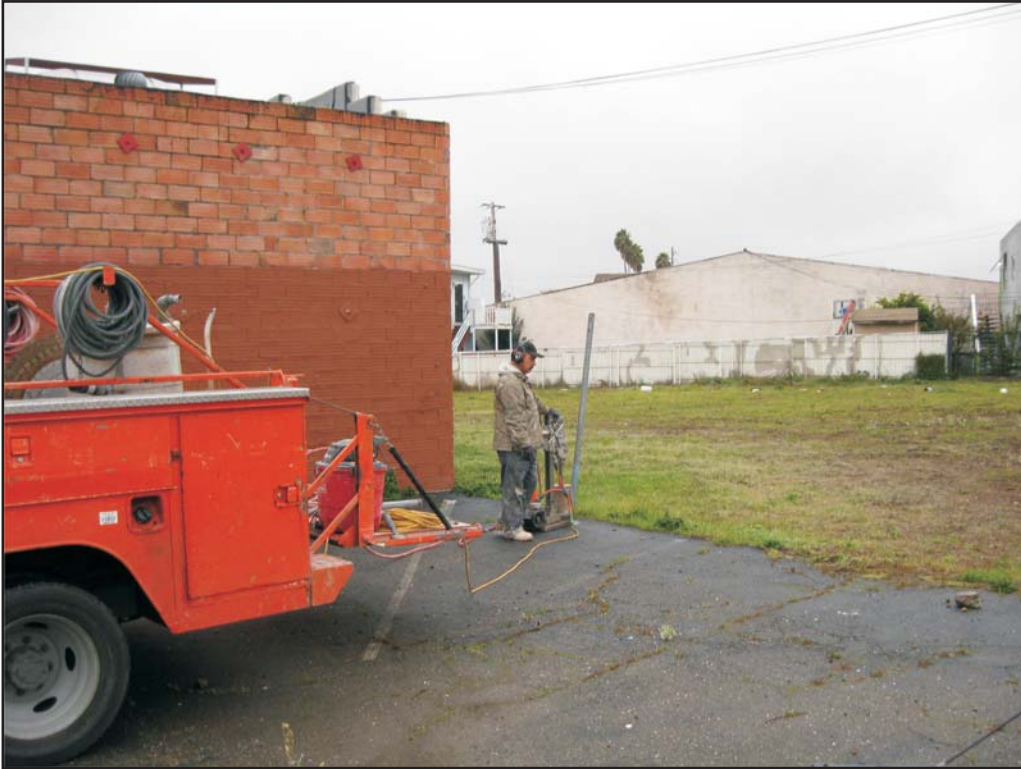
Photograph 3: Cal West coring through asphalt on the former parking lot.
