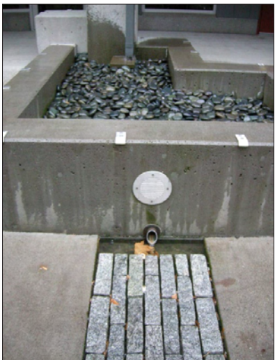
► Figure 3.11.b: This facility gathers rooftop runoff and funnels it to a ground level water feature before it reaches the storm drain system, slowing and filtering the flow.
