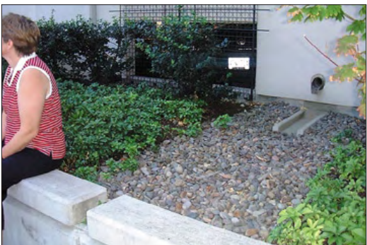
► Figure 3.11.g: The flow-through planter provides seating along the sidewalk and a planting buffer next to the building.
