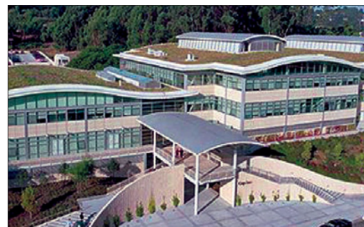
► Figure 3.11.e: This office building in San Bruno is an example of an extensive green roof.
