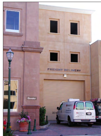
► Figure 3.6.d: Integrated into the building envelope, this one-way loading facility exits on the other side of the building, minimizing its impact on the street.
