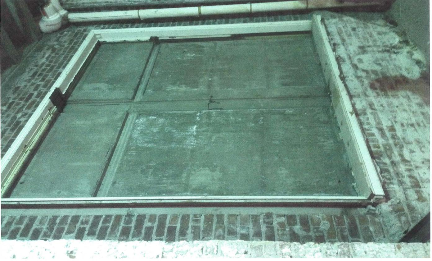
**INTERIOR VIEW OF EXISTING WINDOW OPENING COVERED BY SHOTCRETE**
