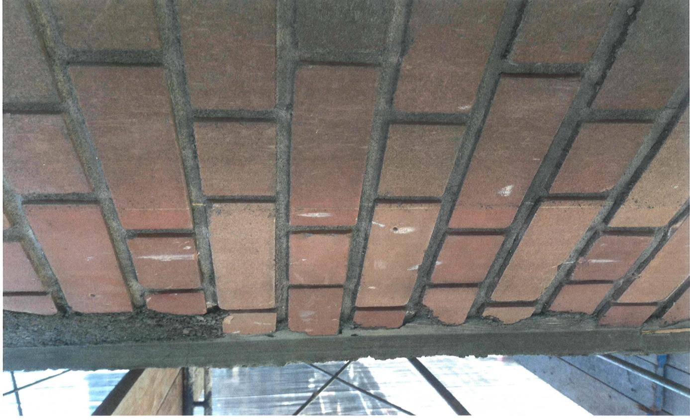
**DAMAGED BRICK AND EXTENT OF SHOTCRETE AT CORNER**
