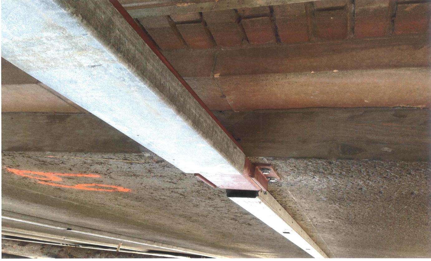
SHOTCRETE OVER BRICK AND CHANNELS THROUGH TERRA COTTA PILASTERS
