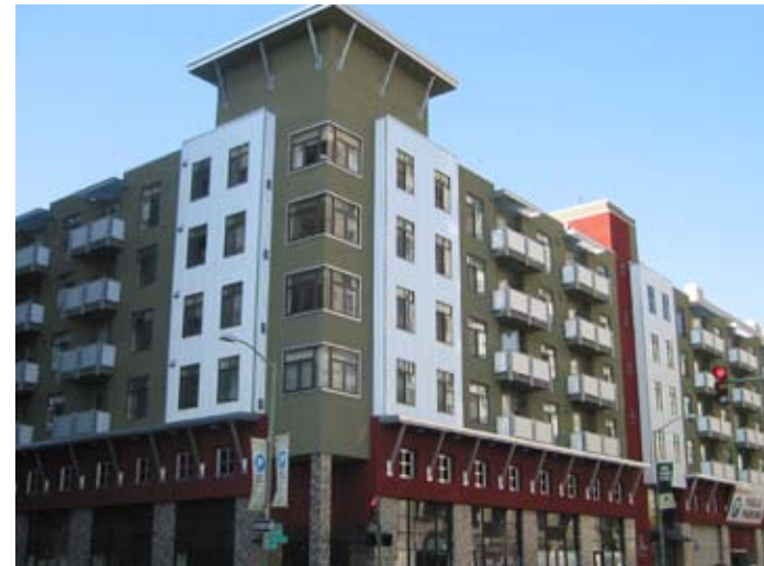
New housing development in Chinatown.
