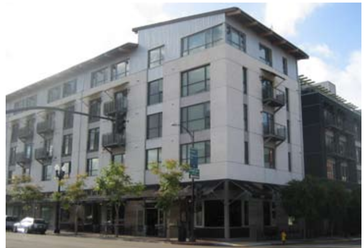
Residential above ground-floor retail
