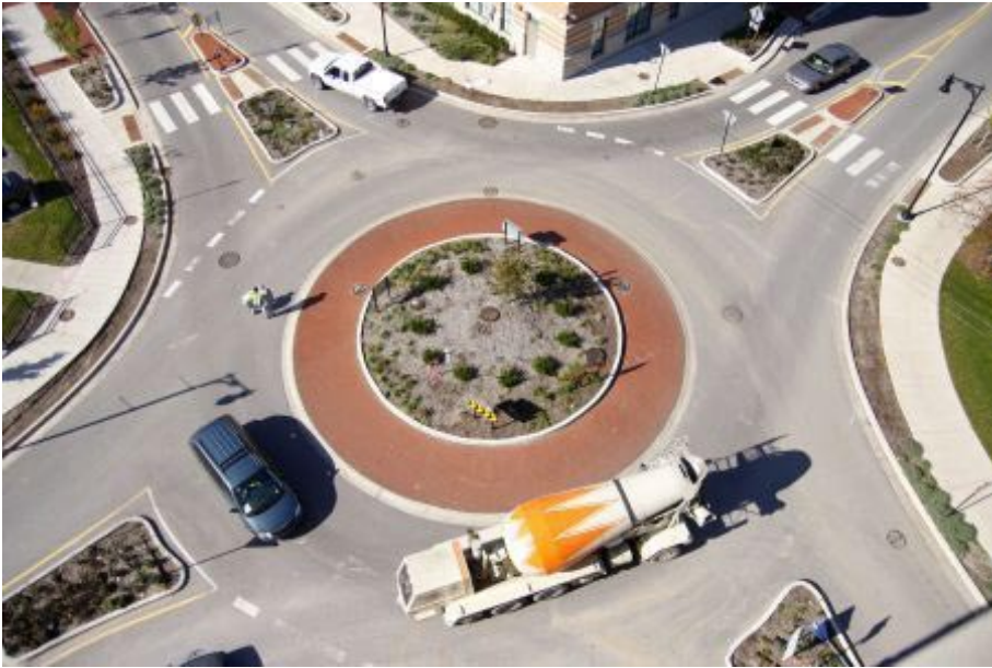
Large vehicles easily pass through roundabouts
