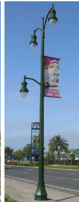
High-low tear-drop lighting for sidewalk and street
