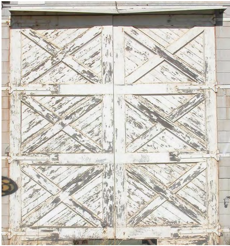
Figure 4.35. Door detail, Building 991. Each door has three cross-braced panels with diagonal sheathing.
