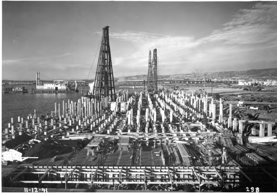
Figure 3.1. Driving concrete piles for the base's east wharf (Wharf 6), adjoining the old Union Construction shipyard, November 1941. (Port of Oakland Archives.)
