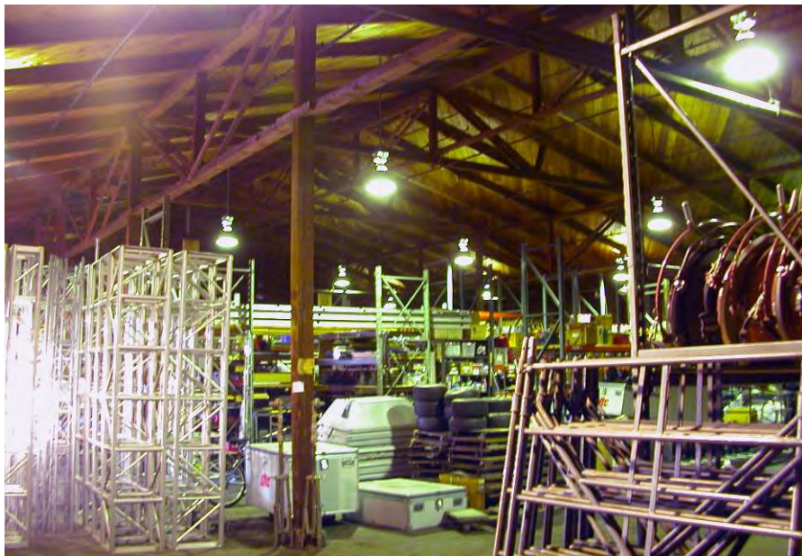
Figure 4.30. The heavy timber construction of Building 821 consists of two rows of timber posts supporting flat and gabled trusses.
