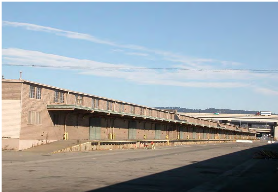
Figure 4.20. South side of Building 806. Elevated loading docks with canopies extend along both sides of the “800 series” warehouses. Each dock is served by 17 doorways, or loading bays, with sliding wood doors. Rows of paired wood-sash windows surmount the canopies.
