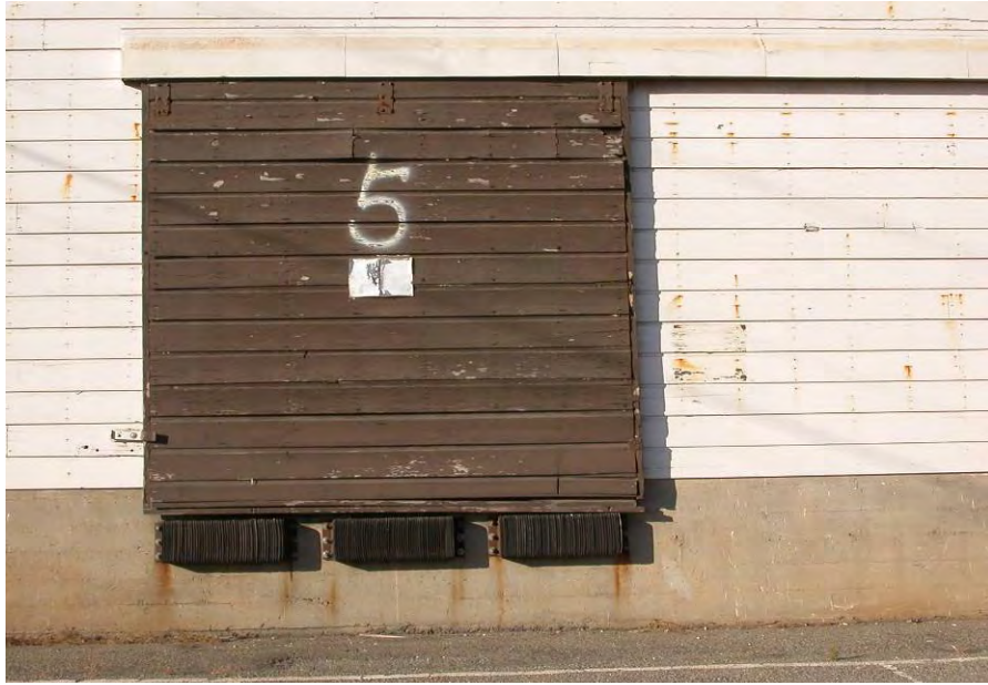
Figure 3.11. Exterior-mounted, sliding wood door on south side of Building 821. Five such doors are hung along each side of Buildings 821 and 822. Note the horizontal wood siding, which is wider than that on the “800 series” warehouses.
