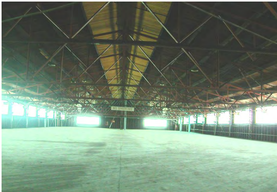
Figure 4.15. Former mold loft, Building 99. Spanned by steel trusses, this spacious room is encompassed by windows and capped by a skylight, now covered with translucent plastic. The floor is laid with diagonal boards.
