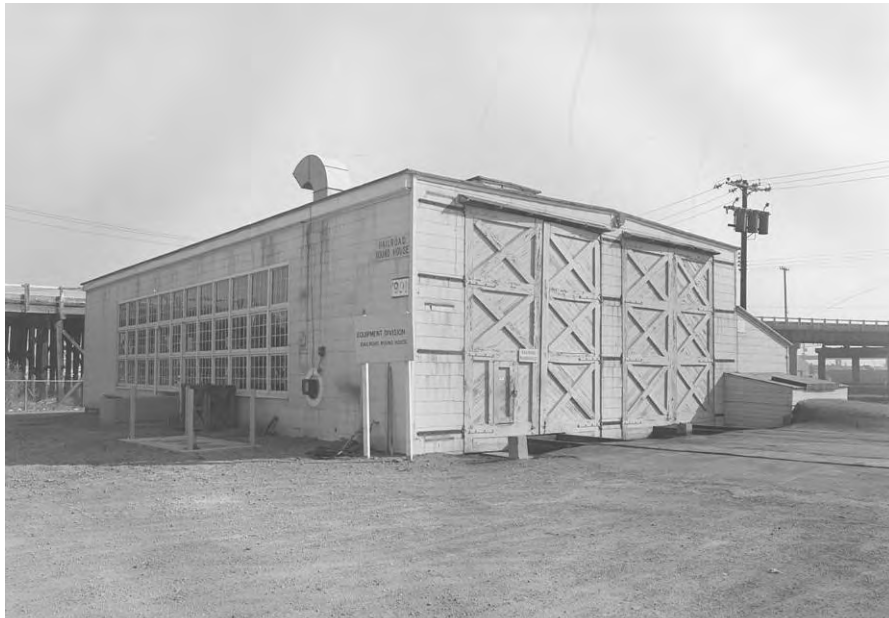
Figure 4.33. Building 991, perspective view looking east, 1976. Built in 1942 in conjunction with the Knight Rail Yard, this building served as the base's repair and maintenance facility for locomotives. It was known variously as the Engine Switch Shop, Railroad Engine Shop, and Railroad Roundhouse. Spur tracks led from the rail yard to the shop, branching to enter two service stalls served by tall hinged doors. (Oakland Army Base Archives.)
