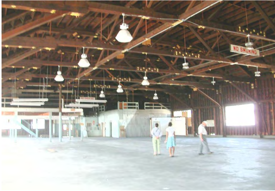
Figure 4.9. Massive timber trusses form a clear span in Building 88. This view also shows the partitioned rooms and mezzanine floors added at the south end of the building, occupying a small fraction of the interior space.
