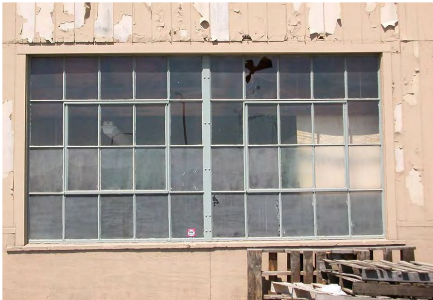
Figure 3.18. Steel-sash window, Building 88. The Port of Oakland’s reconstruction of this World War I-era building probably included the addition of steel-sash windows, although they may form part of the original structure. Because of restrictions on the use of steel, all World War II-era buildings on the base have wood-sash windows.
