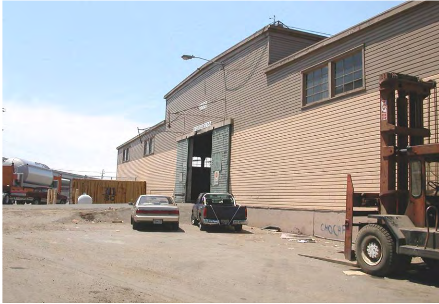
Figure 4.21. Building 808, east end. This view shows the central bay, with monitor, and flanking side bays. Note the ramped entry with sliding wood doors, as well as the wood-sash windows (limited to the upper level at this end of the building). The exterior is uniformly clad in horizontal wood siding.
