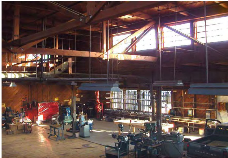
Figure 4.32. The heavy timber construction of Building 823 features large monitor trusses spanning the central bay. Note the diagonal board sheathing on the partition and sidewall.
