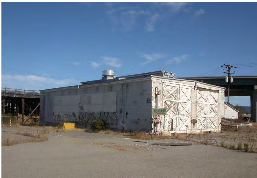
Figure 4.34. The building is largely intact. Asbestos-cement shingles have been added over the wood siding of the walls, and sheets of plywood cover the large window panels.
