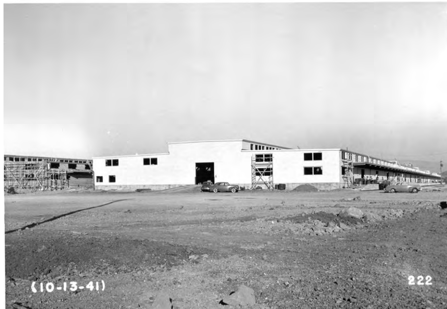
Figure 4.17. This early view, looking east, depicts one of the “800 series” warehouses (probably 802) nearing completion in October 1941. The wood siding has been painted, but windows and doors are not yet installed. Framing and sheathing is in process on the warehouse to the left. (Port of Oakland Archives.)
