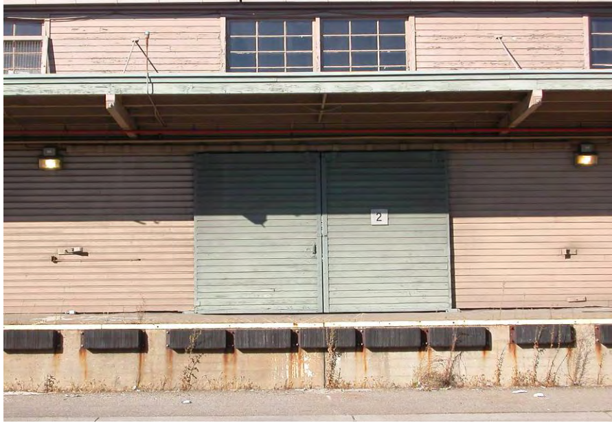
Figure 3.9. Doors on south loading dock, Building 806. Each of the “800 series” warehouses has 17 identical freight-handling bays arrayed along each side of the building. This representative view shows the exterior-mounted, sliding wood doors, clad in horizontal wood siding to match the exterior cladding of the walls. Note the fixed-pane, wood-sash windows over the canopy.
