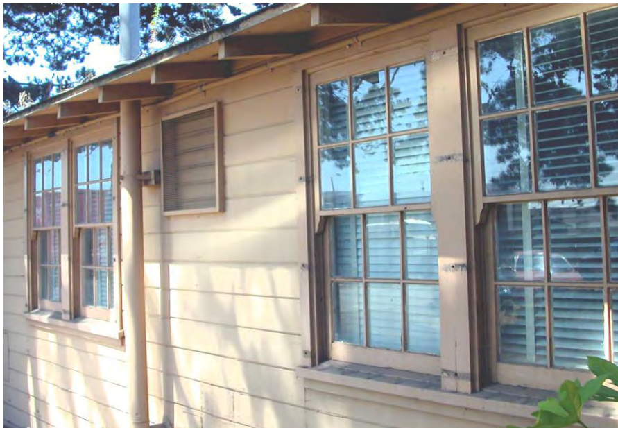
Figure 3.16. Similar six-over-six double-hung windows can be found on Building 90, though most windows on this building have been replaced with aluminum sash.
