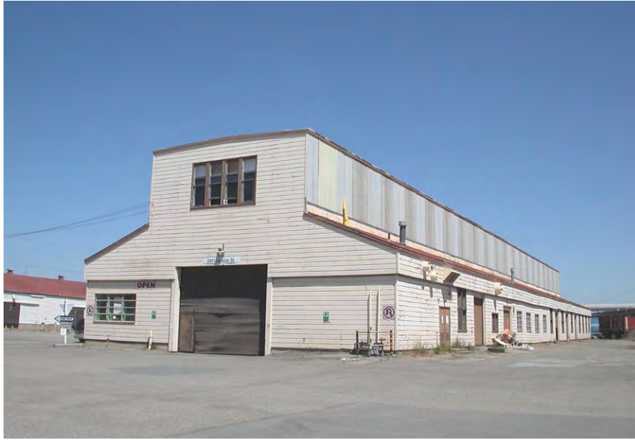
Figure 4.25. Building 812, perspective view of west end and south side. The most prominent feature of the building—a bulky monitor accommodating a rolling bridge crane—has been altered by the application of asbestos and fiberglass panels.
