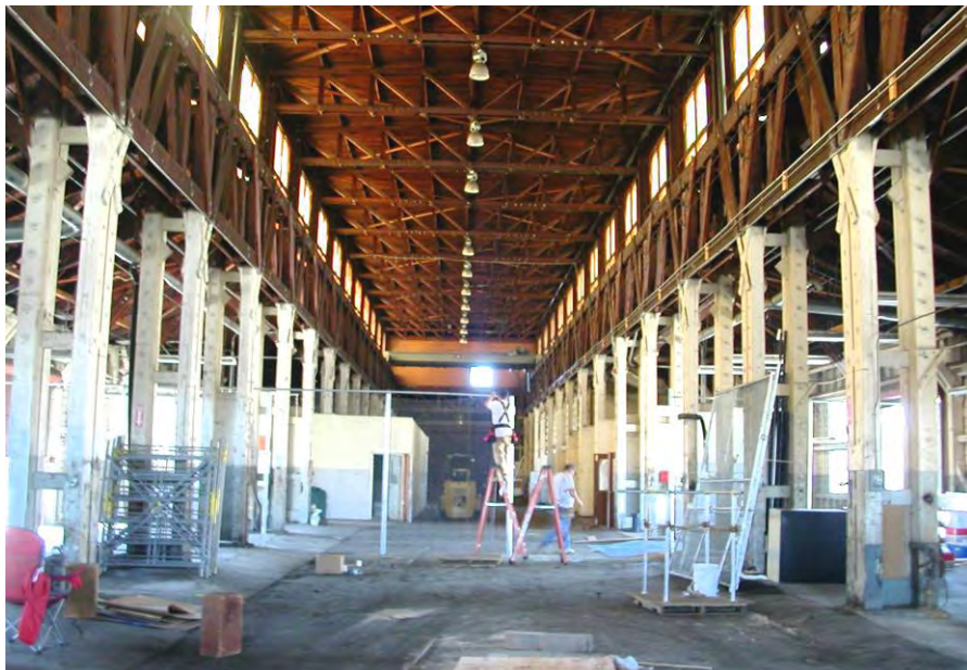
Figure 4.28. The double rows of heavy timber posts support truss-work rails serving a 5-ton rolling crane (visible in distance).
