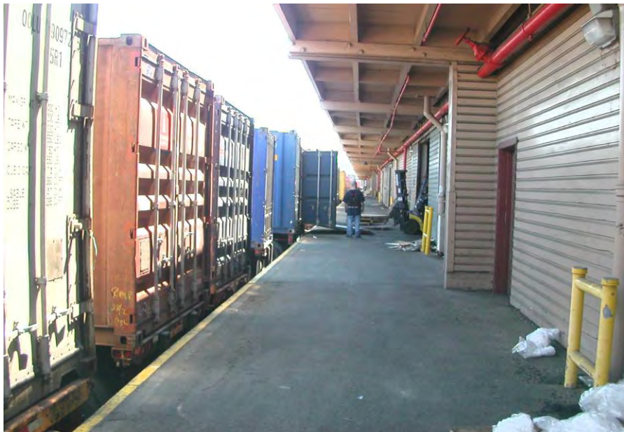
Figure 4.22. Building 808, north loading dock. This view highlights the cantilevered form of the canopy and the horizontal wood siding of the walls.
