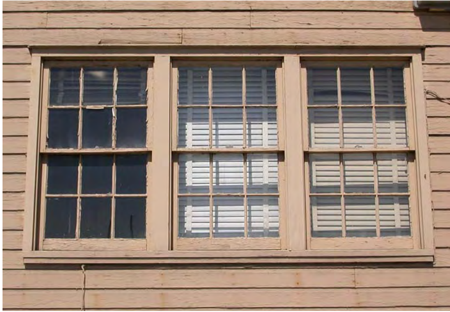
Figure 3.15. Multi-light, wood-sash windows survive in most buildings on the base, including more than 40 double-hung windows on Building 85.
