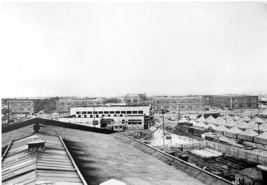
Figure 3.4. In this similar view, taken from the roof of Building 99 five weeks later, in early December, the Administration Building and Cafeteria have been enclosed with diagonal board sheathing. The tents may be those of the 394 th Quartermaster Battalion, an African-American unit that assisted in the first phase of construction at Oakland Army Base. (Port of Oakland Archives.)
