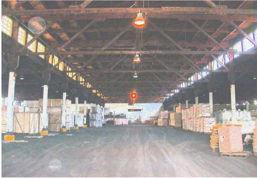
Figure 4.23. Building 808, interior view of central bay. Wood trusses on heavy timber posts support the wide, window-lined form of the monitor.
