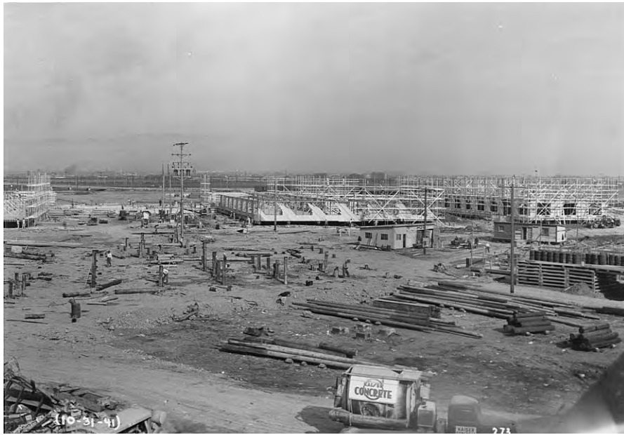
Figure 3.3. Construction activity at Oakland Army Base, October 1941. In this view (looking north from Building 99), the wood frame of the Administration Building is going up, with diagonal wood sheathing partially in place. The filled land required piles to support foundations, and numerous timber piles are visible stacked on the ground. Workers can be seen around the piles that have been driven for the Cafeteria (Building 60), at left-center of image. (Oakland Army Base Archives.)
