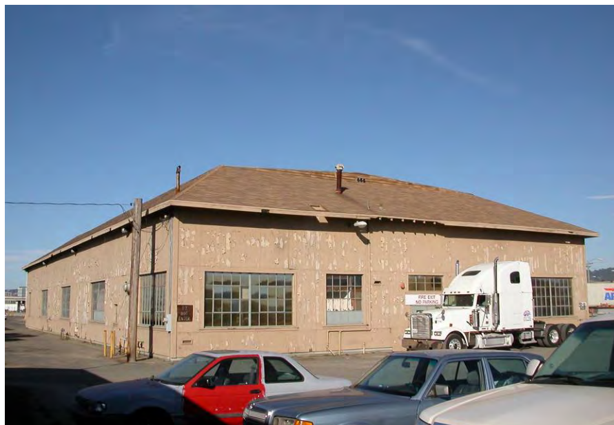
Figure 4.8. This view looking northeast shows the veneer of vertical wood paneling that has been applied over the original horizontal wood siding of Building 88, as well as the steel-sash windows dating from World War I or the 1930s. The original doorway at south end of the building has been enclosed; the doorway at the north end is intact.
