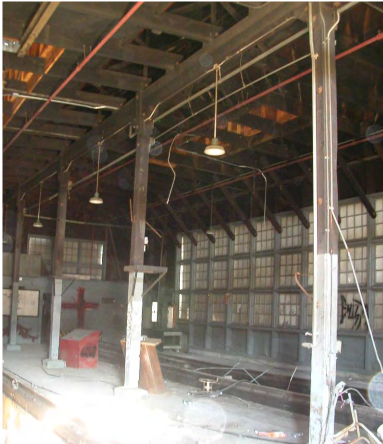
Figure 4.36. Building 991's two service bays (one equipped with a pit) are separated by a row of heavy timber posts running down the center of the floor, with several small partitioned rooms and a mezzanine at the far end. Note the intact window panels at the side and rear.
