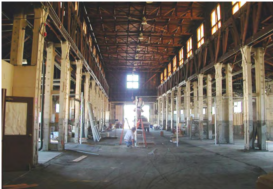
Figure 3.8. Heavy timber construction, Building 812. The double rows of bolted timber posts support longitudinal, truss-work rails for an overhead crane as well as the elevated structure of the monitor, incorporating transverse roof trusses.
