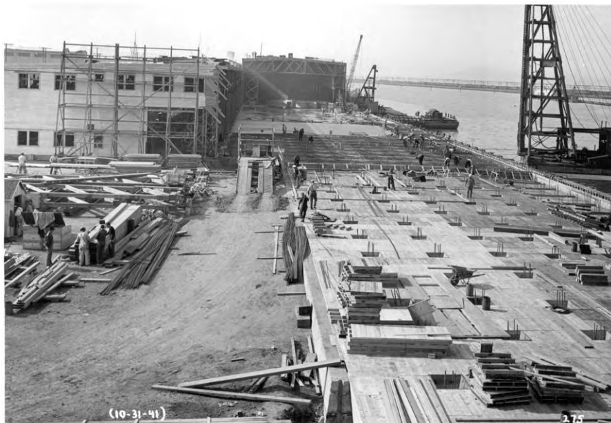
Figure 3.2. Construction underway on the south wharf and transit shed, October 1941. Note the tops of the regularly spaced concrete piles, providing support for decking and floors. (Port of Oakland Archives.)
