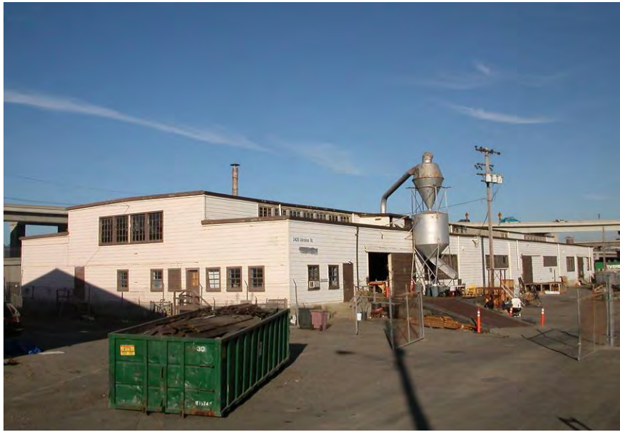
Figure 4.31. Building 823, perspective view looking east. Though quite similar to Buildings 821 and 822, this former box factory was built a year earlier, in 1942, and incorporates a monitor in its design.
