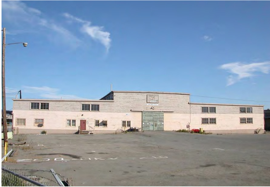
Figure 4.19. West façade, Building 804. The tripartite form of the “800 series” warehouse is clearly seen in this representative view showing the wide central monitor flanked by lower side sections. Windows provide light on two levels; sliding wood doors serve the doorway.
