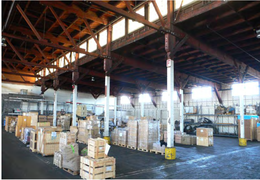
Figure 3.7. Heavy timber construction, Building 808. The “800 series” warehouses utilize grids of timber posts to support the timber girders of the side bays and timber trusses in the central monitor.
