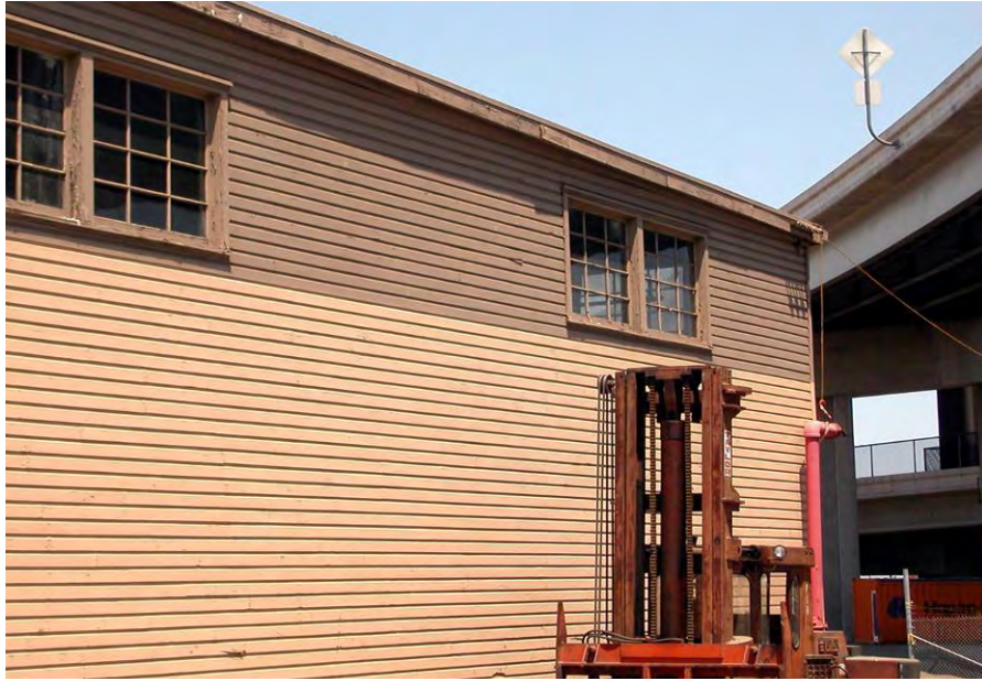
Figure 3.17. Building 808, east end detail. Multi-light, fixed-pane, wood-sash windows are set into the walls at each end of the “800 series” warehouses as well as in rows above the canopies and along the monitors. This view also shows the generally good condition of the exterior wood siding on these buildings.
