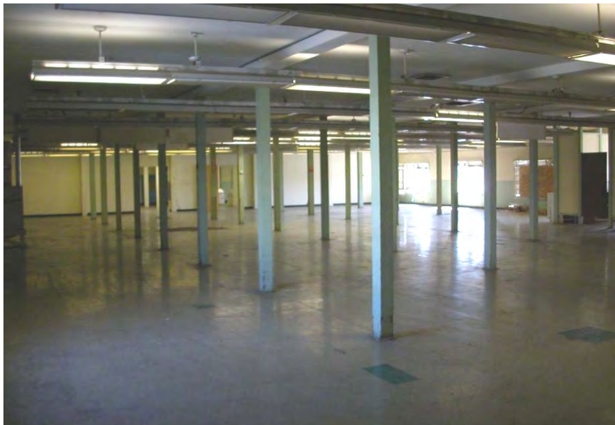
Figure 4.6. Alterations to the interior of Building 85 include linoleum flooring, plasterboard walls, a dropped ceiling, and modern light fixtures. The timber posts are original.
