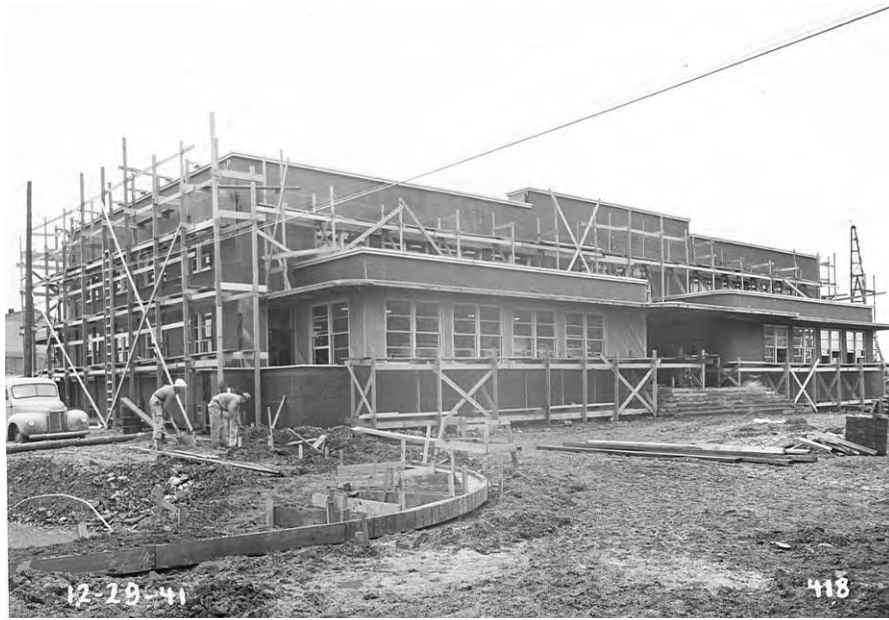
Figure 3.5. Close-up view of the Cafeteria (Building 60), looking west, late December 1941. The building is receiving a veneer of stucco over the diagonal board sheathing. (Oakland Army Base Archives.)
