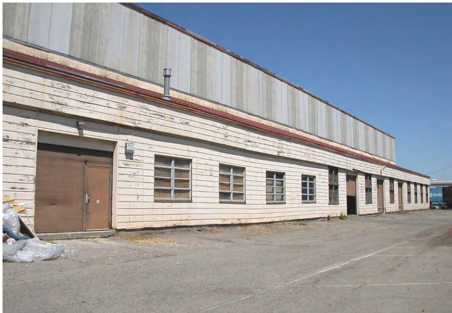
Figure 4.26. Building 812, south side. Most windows have been replaced with aluminum sash, and sliding wood doors have been replaced with roll-up metal doors. Walls retain the original horizontal wood siding.
