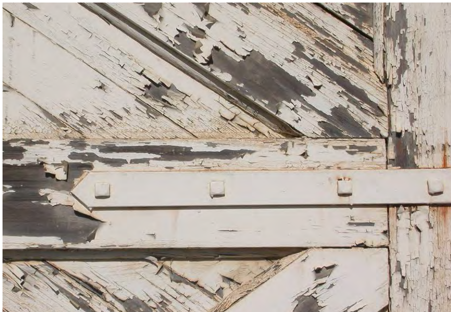
Figure 3.12. Door detail, Building 991. The two pairs of hinged wood doors on the railroad roundhouse have diagonal sheathing and bolted iron strap hinges.
