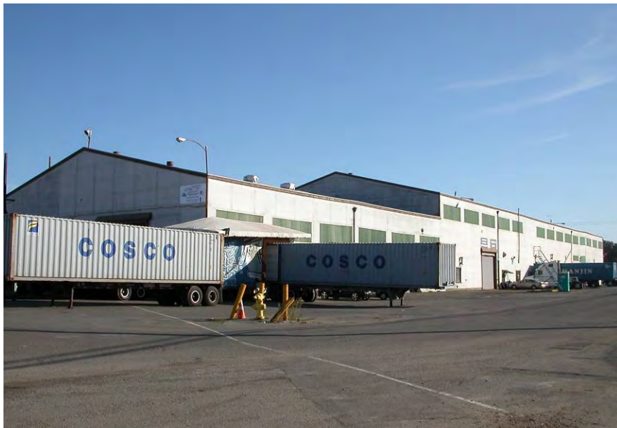
Figure 4.14. Building 99, looking southwest. This view clearly shows the scale and the stepped, gabled massing of the structure. The exterior has been altered by the application of asbestos-cement panels over the original horizontal wood siding and the enclosure of windows with translucent plastic panels.
