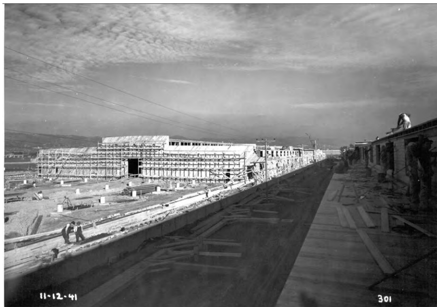
Figure 3.6. Looking east to warehouses under construction, November 1941. One or more sections remain to be built on the warehouse to the left. The exposed firewall partition, with diagonal board sheathing, is covered with scaffolding, and concrete footings are in place for the floors of the next section. The forms for the concrete loading dock are being inspected by two workmen (lower left), and workers (right) install windows atop the loading-dock canopy on the warehouse in shadow. (Port of Oakland Archives.)
