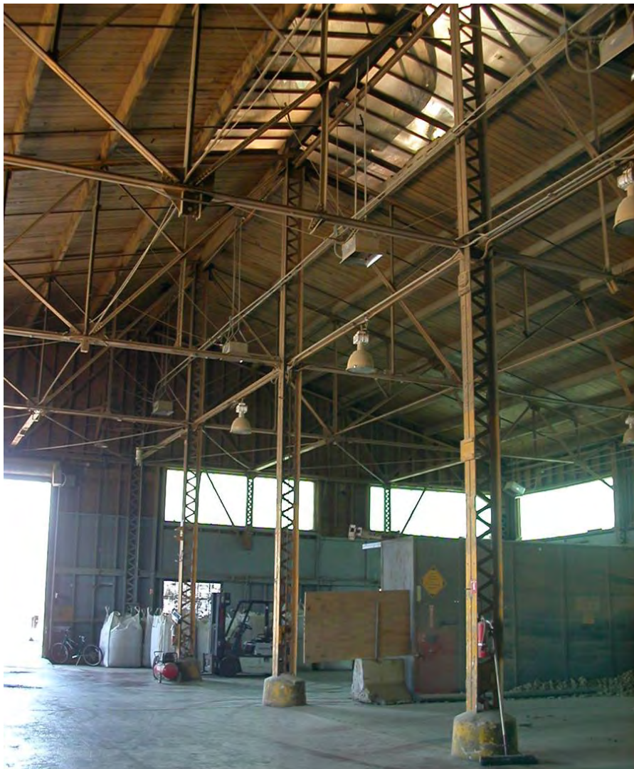
Figure 4.16. Building 99 is the only steel-frame structure in the Oakland Army Base Historic District. This view shows the trussed steel columns and spindly trusses of the one-story section at the north end of the building.
