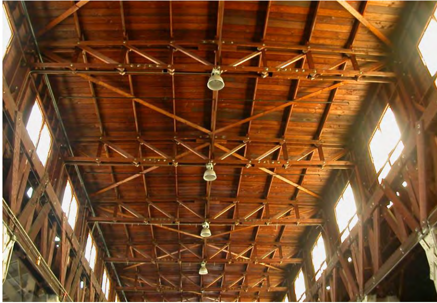
Figure 4.27. Building 812, interior view of monitor. Bolted wood trusses and purlins support the roof decking.
