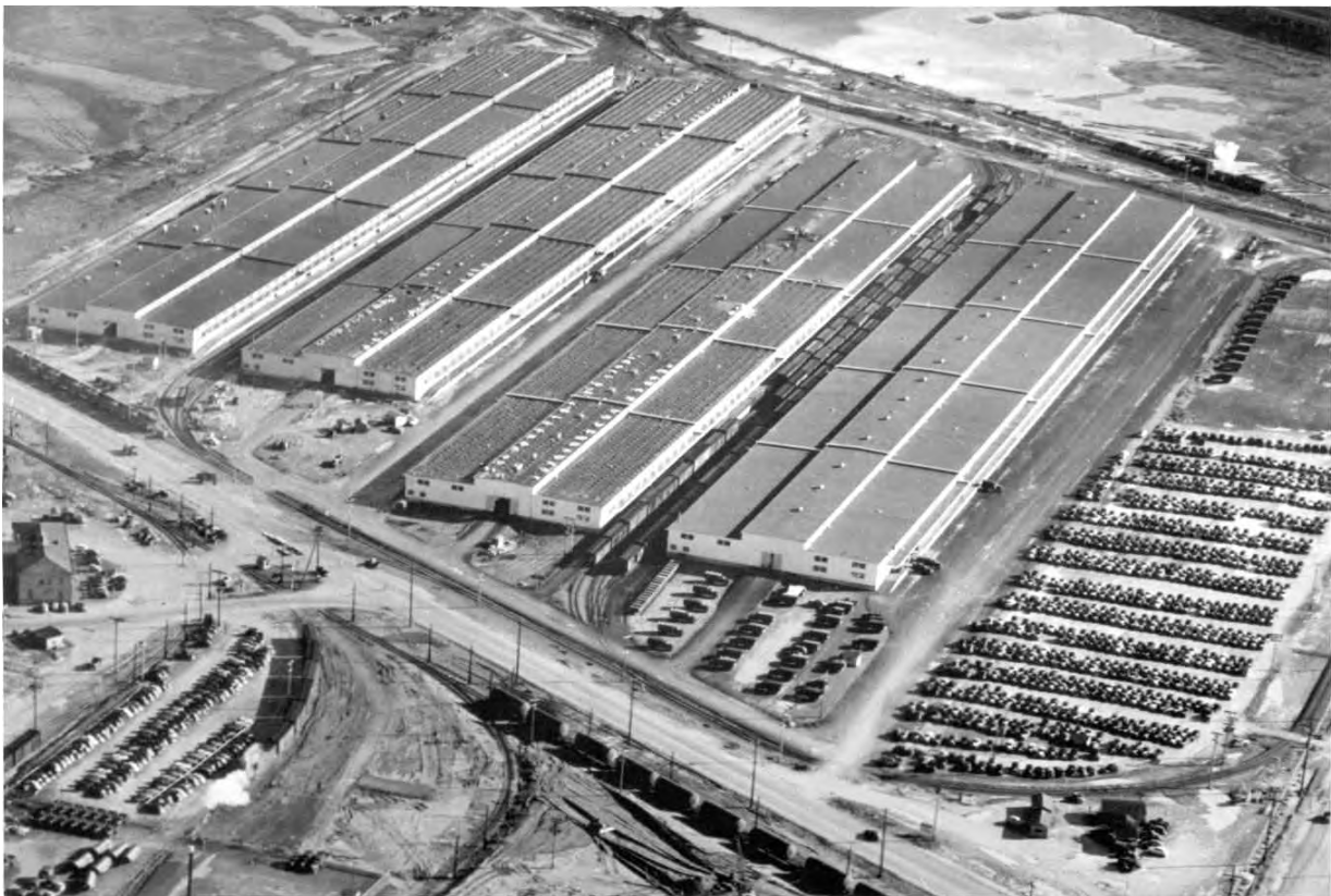
Aerial View of the "800 Series" Warehouses in mid-1942. The warehouses shown (from right to left) are Buildings 802, 803, 804, and 805. The final three warehouses in the row (Buildings 806, 807, and 808) were completed later that year. (Source: Port of Oakland Archives)
