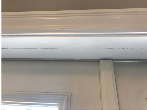
Photo 16: French Door Interior water intrusion
