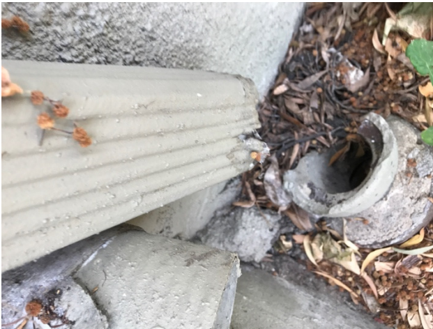
Photo 8: Clay drainage appears to be original
