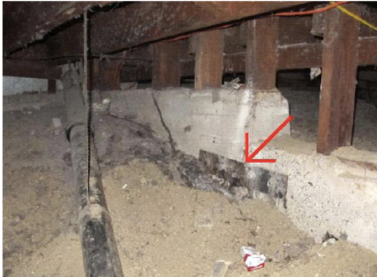
Photo 4: Crack covered by steel strap and spalling
