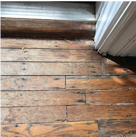
Photo 17: Interior wood damage from water intrusion issues associated with French door
