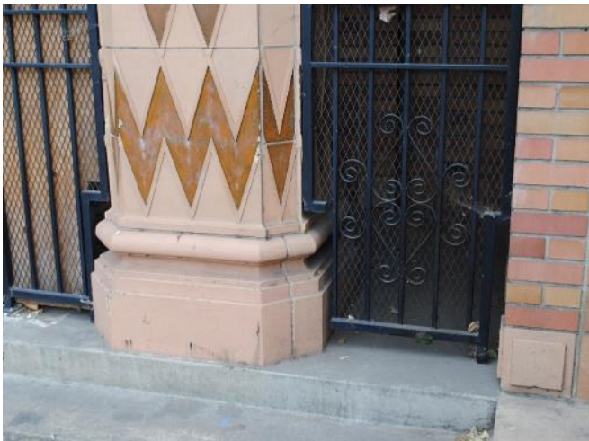
Replacement of iron grill at main entry with more compatible design. Removal or damage of original terra cotta and brick materials will be avoided during the removal and installation of the new grill.
