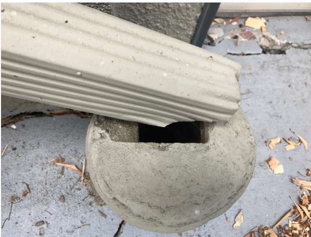
Photo 9: Clay drainage appears to be original
