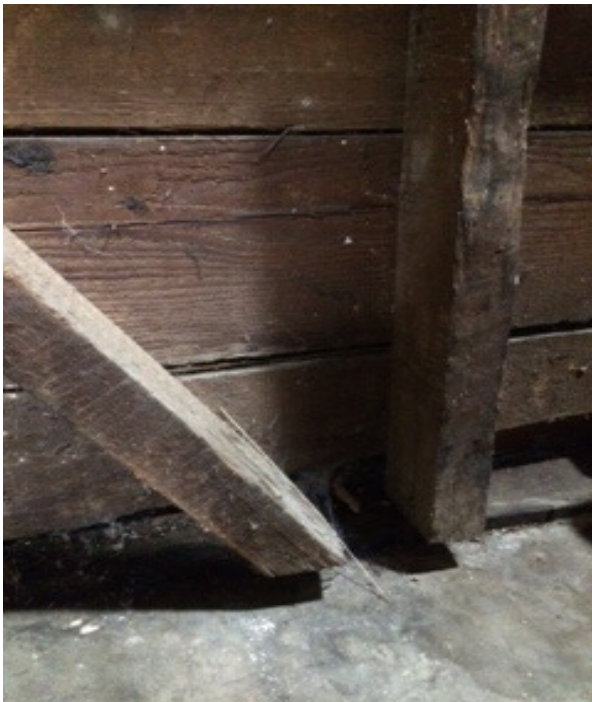
Garage separating from foundation
