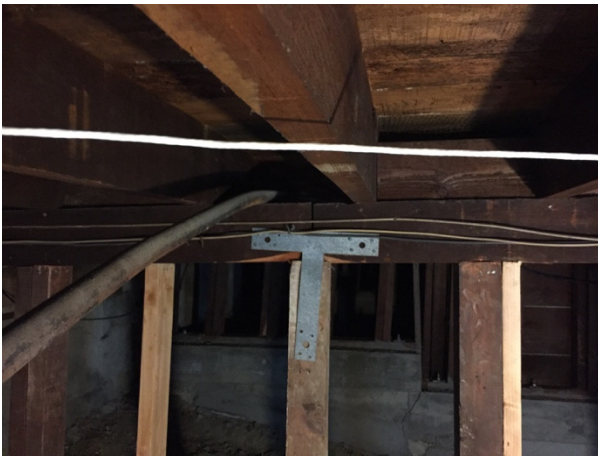
Photo 2: Tilting cripple studs and brace (racked framing)
