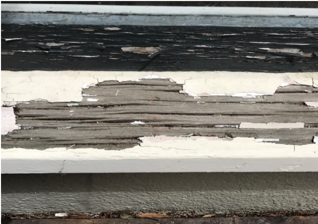
Photo 12: Sill damage on center picture window
