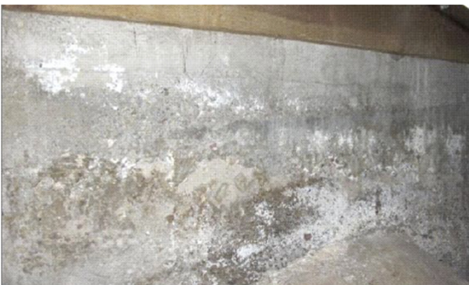
Photo 10: Efflorescence at foundation wall
