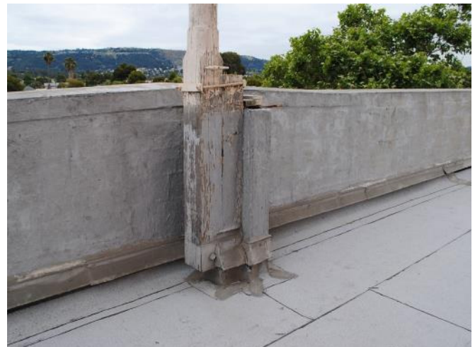
Restoration of flagpole, including counter-flashing at roof.
