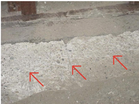
Photo 5: Cracking and spalling
