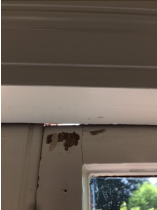
Casement window details of gap and rot
