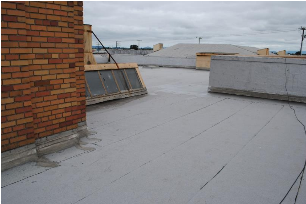
Counter-flashing work at tower connection to roof.
