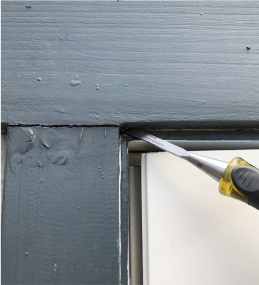
Photo 18: Frame rot on French door
