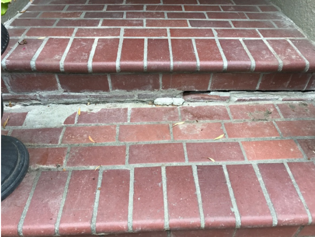
Photo 6: Brick Entrance Stairs Crack
