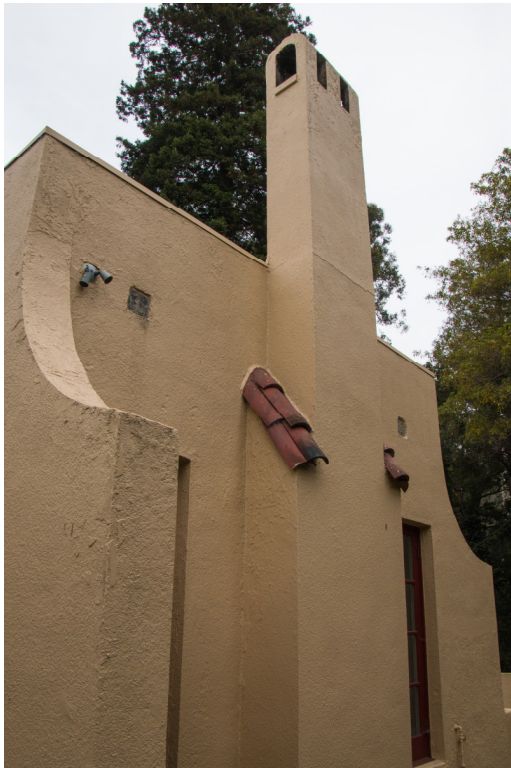
Chimney in danger of collapse
