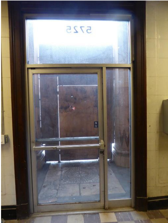
Replace primary entry door and window assembly on primary (north- east) facade with a compatible assembly. View from interior.
