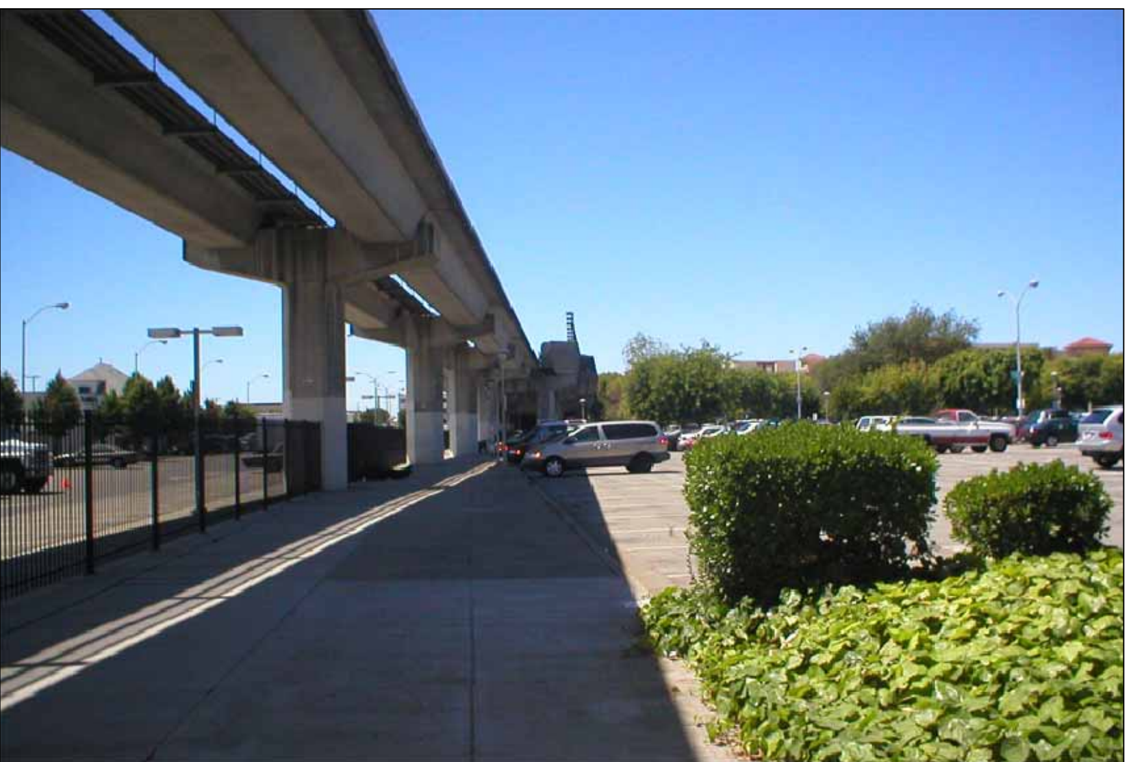
PHOTO #13: FACING WEST ALONG BART TRACKS
