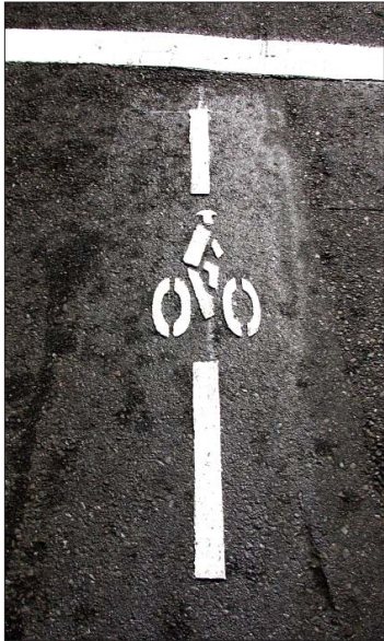
Bicycle detector pavement markings indicate actuated traffic signals that will change for bicyclists.
