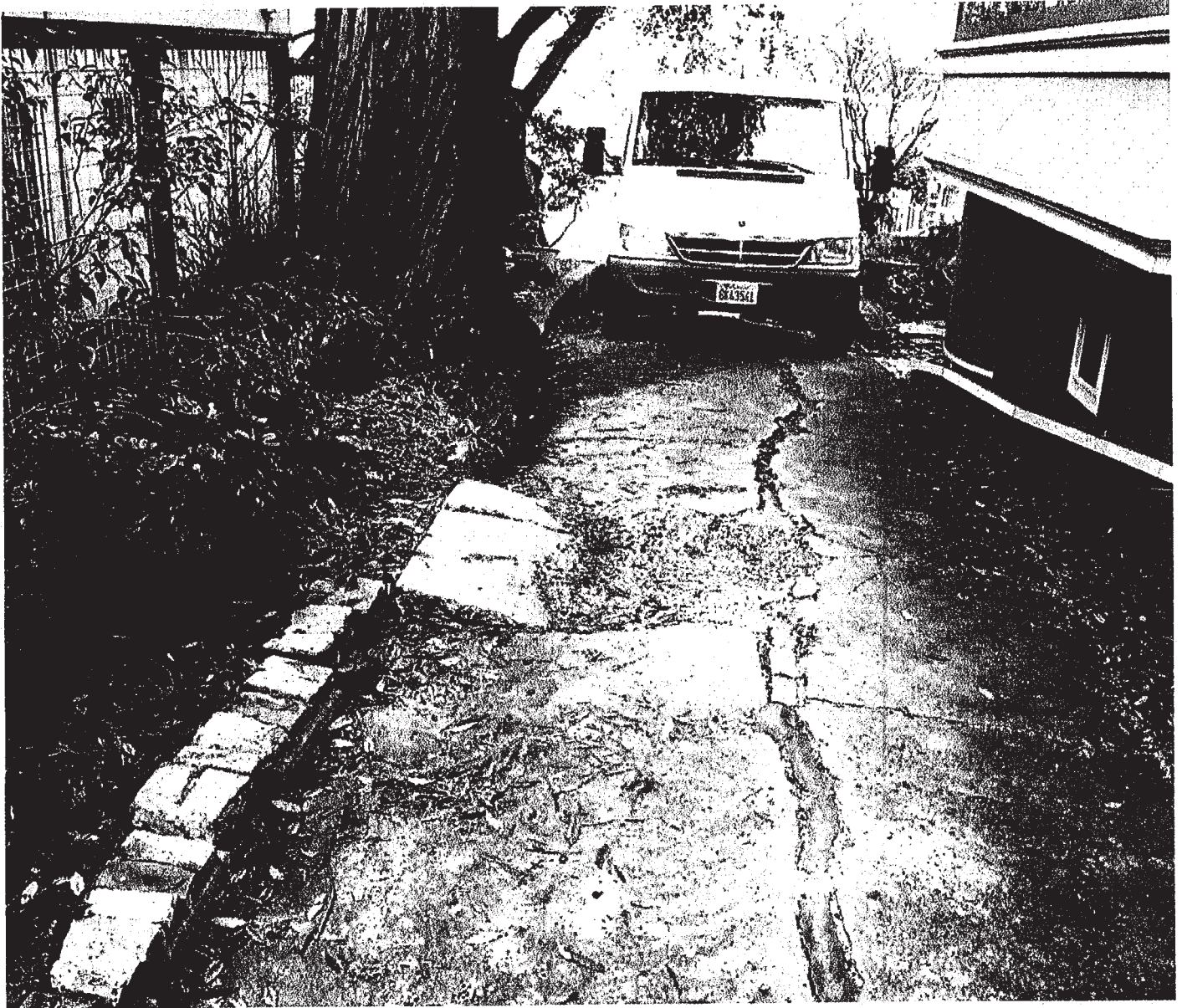
The concrete driveway was cracked, raised up in the center, and depressed next to the tree. There was no apparent damage to the house's foundation, at, or above grade.
